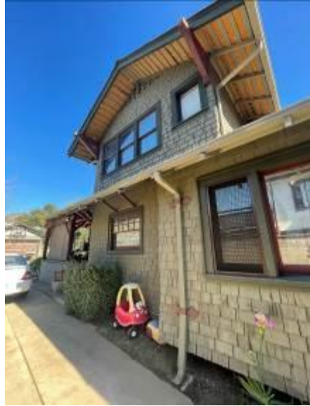
Figure 11. Western Façade SOURCE: Sapphos Environmental, Inc., 2023
