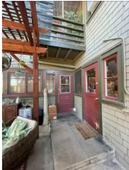
Figure 10. Western Half of the Rear Façade SOURCE: Sapphos Environmental, Inc., 2023
