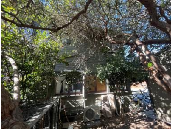
Figure 9. Eastern Half of the Rear Façade SOURCE: Sapphos Environmental, Inc., 2023
