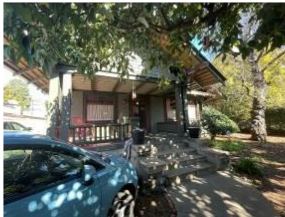
Figure 3. View of the Primary Façade (note the multi-light over one fixed and sash windows) SOURCE: Sapphos Environmental, Inc., 2023
