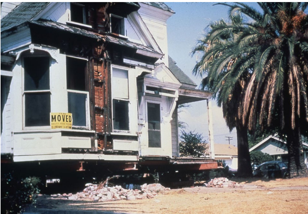
Figure 4 Prepared for relocation, 1980; angled view of incision in center of building; courtesy The Glendale Historical Society
