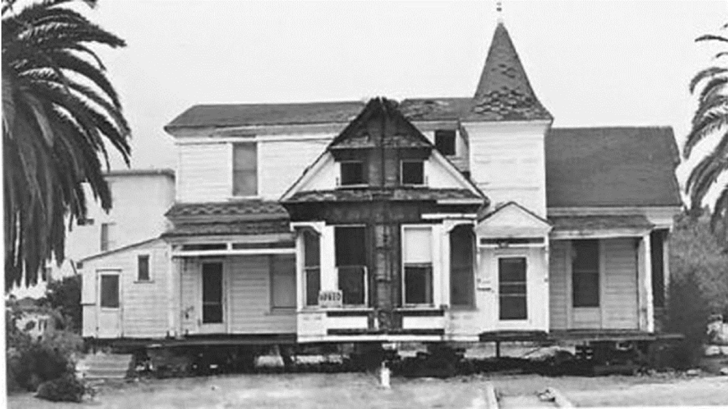
Figure 4 Prepared for relocation, 1980; angled view of incision in center of building; courtesy The Glendale Historical Society
