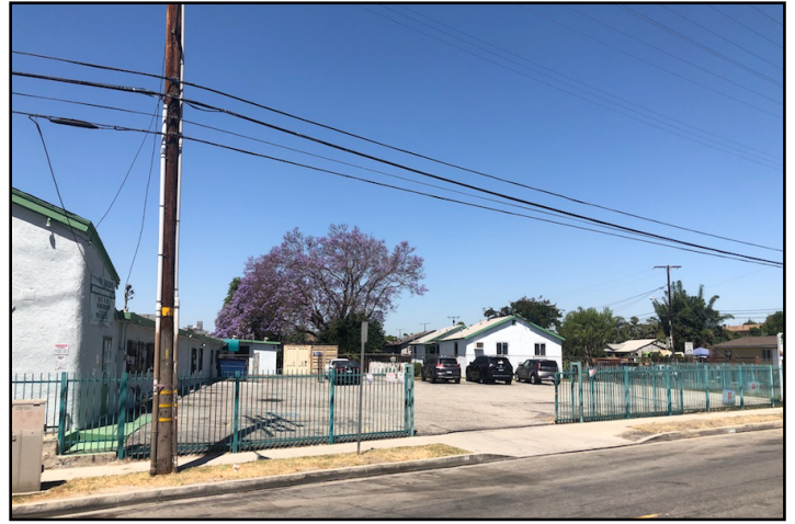
View 2: From the east side of Willowbrook Avenue, looking west at the Project Site.
