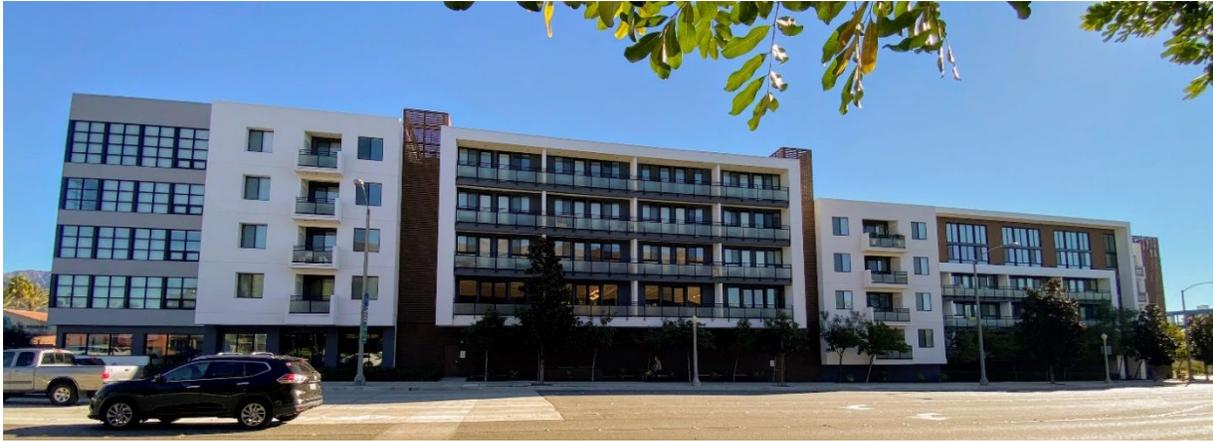
Figure 2-27. Recessed window and offset plane. Source: Gruen Associates
