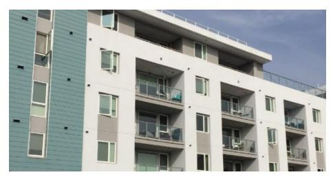
Figure 2-81 Juliette balconies for the top floor units and full balconies for the middle floor units. Santa Monica, CA. Source: Gruen Associates
