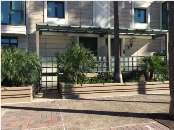
Figure 2-22 Covered patio for ground-floor residential unit adjacent to a public street. San Diego, CA. Source: Gruen Associates
