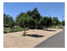
Figure 2-123 High solar reflectance pavers mitigating heat island effect. Governors Island, NY. Source: Gruen Associates
