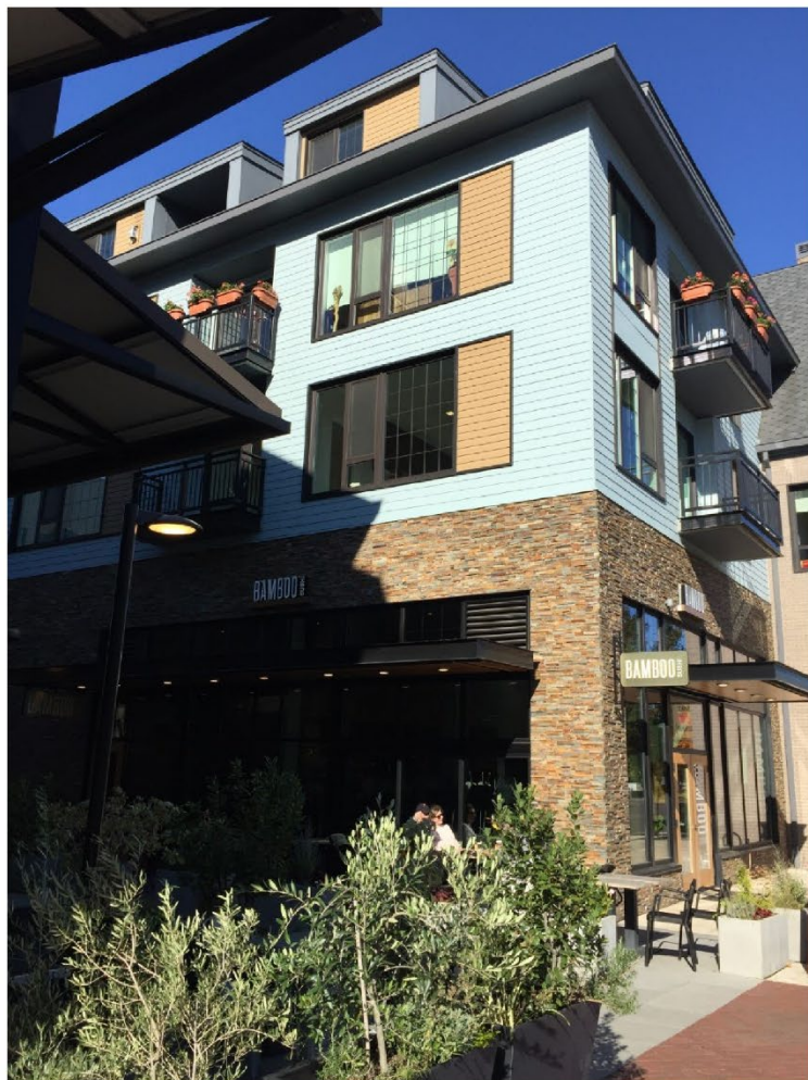
Figure 2-37 Design elements combined to define the base, middle, and top. Lake Oswego, OR. Source: Gruen Associates
