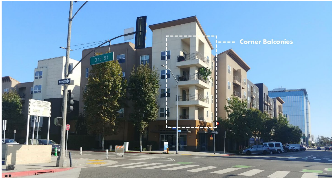
Figure 2-48 Example corner tower with balconies. Long Beach, CA. Source: Gruen Associates
