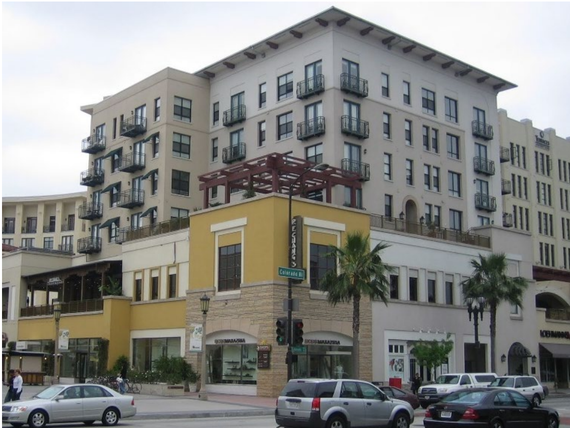
Figure 2-54 Corner of building shorter in height than the rest of the building. Pasadena, CA. Source: Gruen Associates
