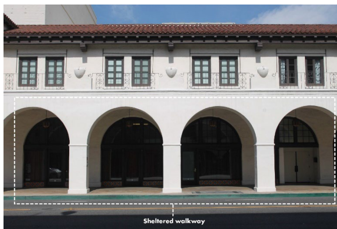
Figure 2-40 Sheltered walkway with horizontal window band, tile roof. Riverside, CA. Source: Gruen Associates
