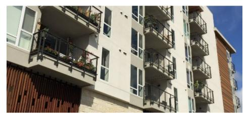
Figure 2-79 Semi-recessed balconies on upper floors. Marina Del Rey, CA. Source: Gruen Associates
