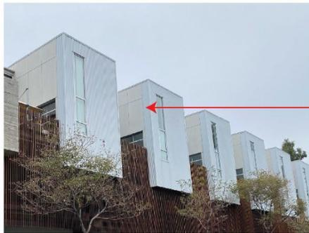
Material wraps around an external corner and ends on the perpendicular wall.
