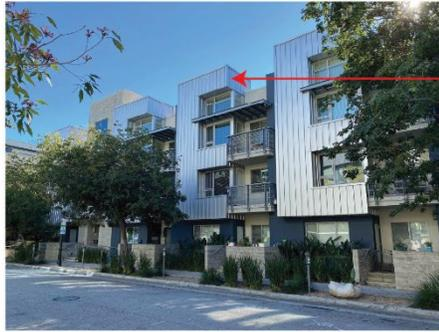
Material wraps around vertical external corner appears integrated into structure.
