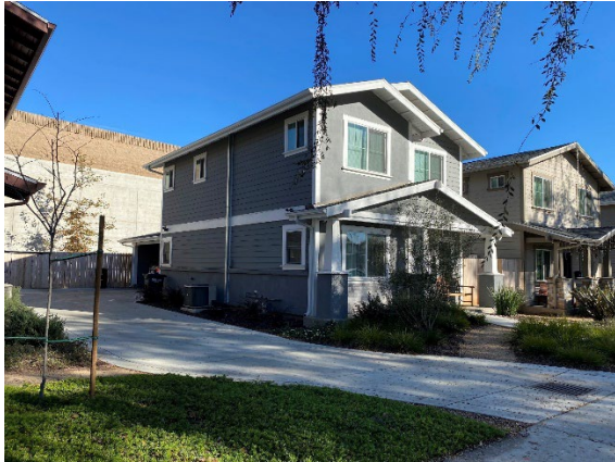
Figure 2-96 Single detached house with parking garage in front occupying 50% or less of the building frontage and recessed behind the porch. Venice, CA. Source: Gruen Associates
