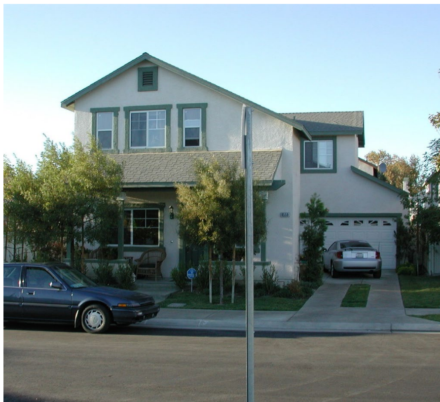
Figure 2-98 Single-unit with garages occupying no more than 50% of the building frontage width and recessed from porch. Portland, OR. Source: Sightline Institute (Flickr.com)
