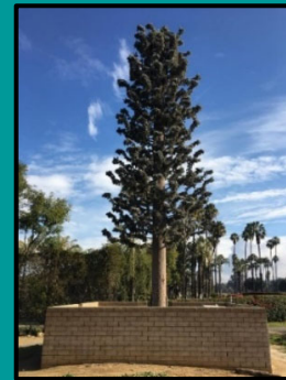
SBA Monarch Towers I, LLC/T-mobile
