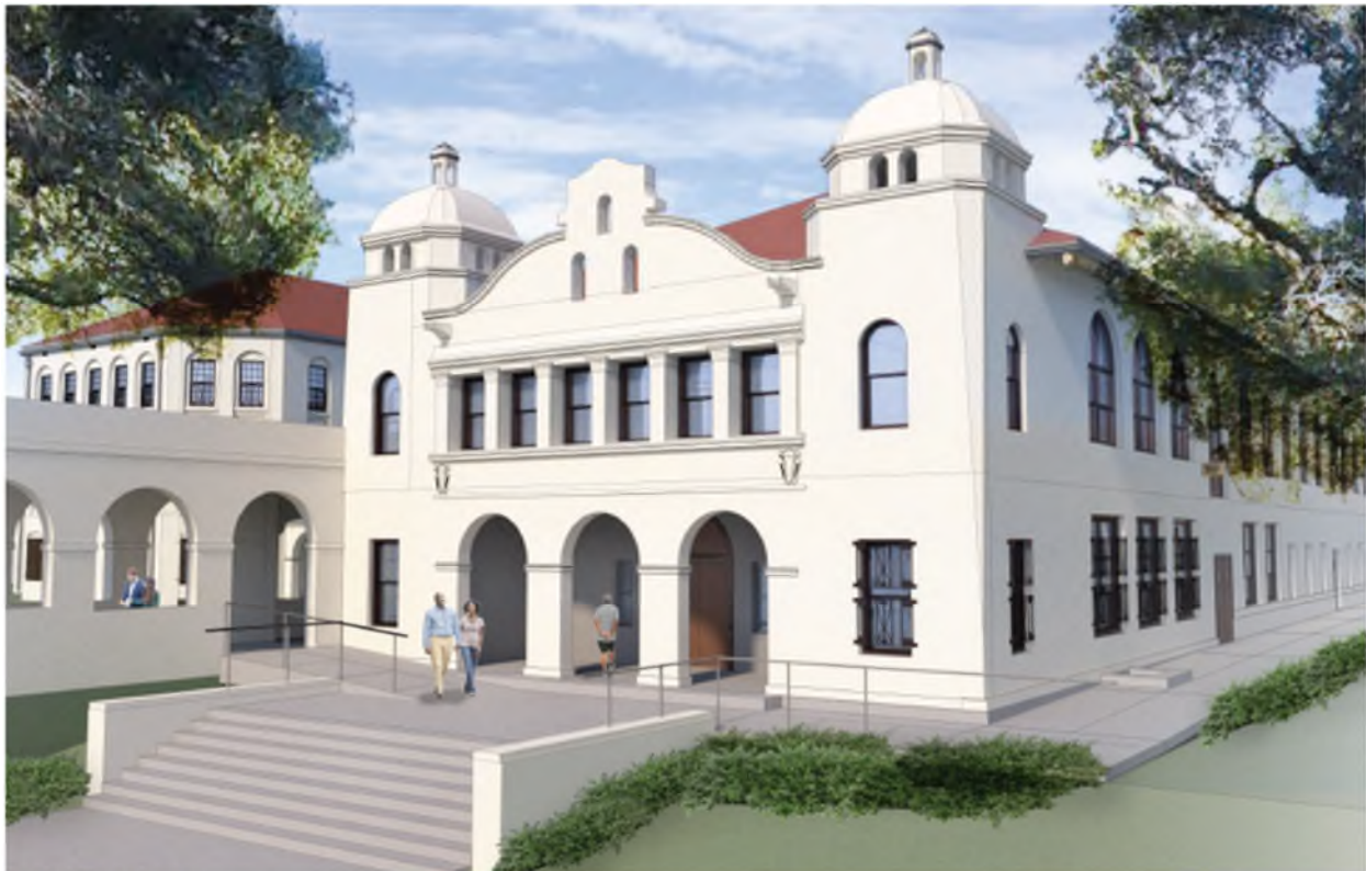
B157 SOUTH EAST CORNER
