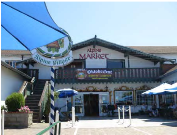
Figure 96. North façade of Alpine Market looking south.
