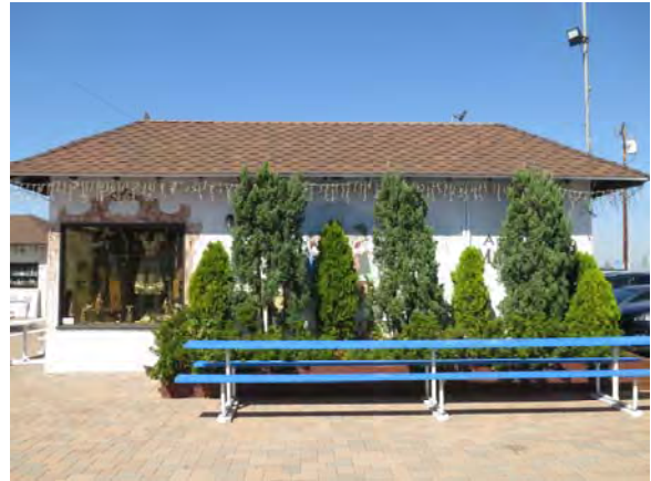
Figure 86. South façade of Building 4 looking north.
