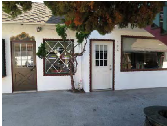
Figure 62. North façade of Building 2 looking south.
