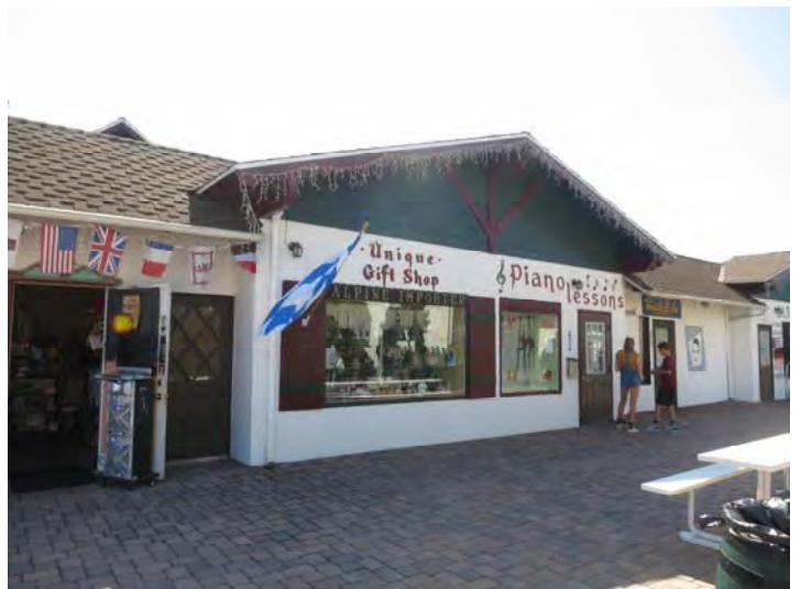
Figure 18. North façade of Building 1 looking southwest.
