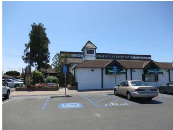
Figure 118. East end of north façade of Alpine Inn.
