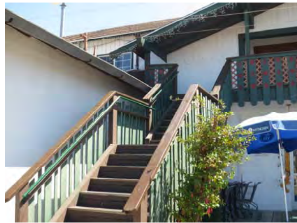
Figure 97. Stairs leading to balcony on north façade of Alpine Market.
