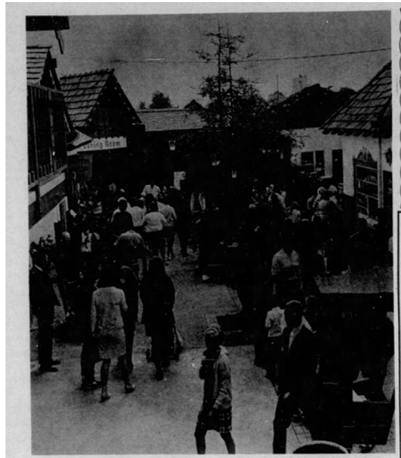
Figure 70. 1971 photo showing restaurant entrance in 1971.
