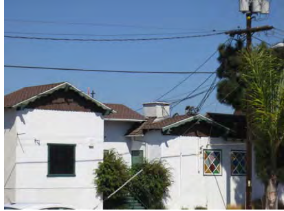
Figure 35. Southwest corner of Building 2.
