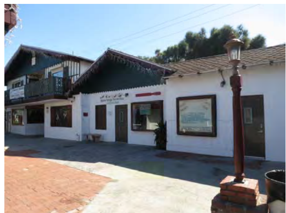
Figure 68. Storefront west of gable on north façade of Building 2.
