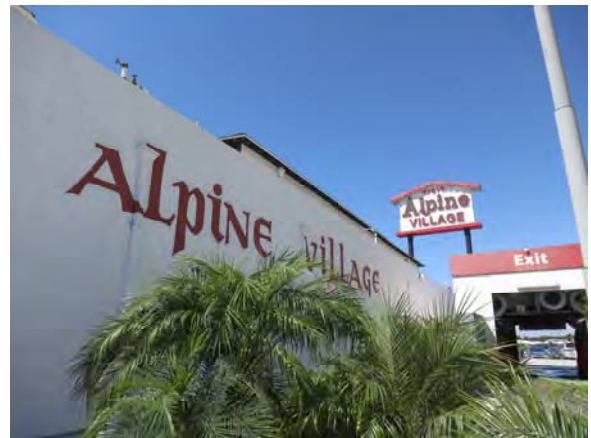
Figure 108. East façade of Alpine Market looking north.
