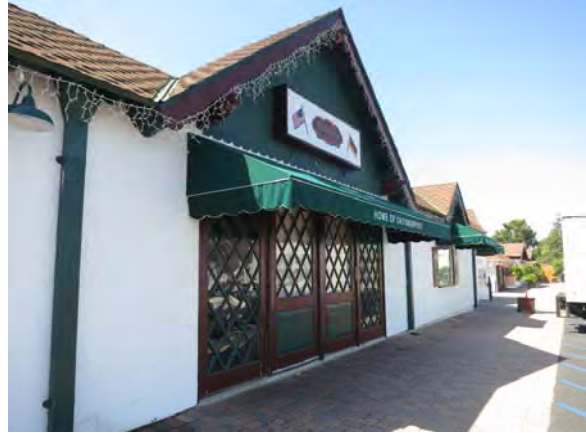
Figure 117. Detail of doors on north façade of Alpine Inn Restaurant.
