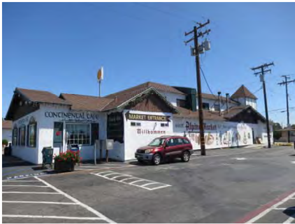
Figure 104. Oblique view of Alpine Market looking southeast.
