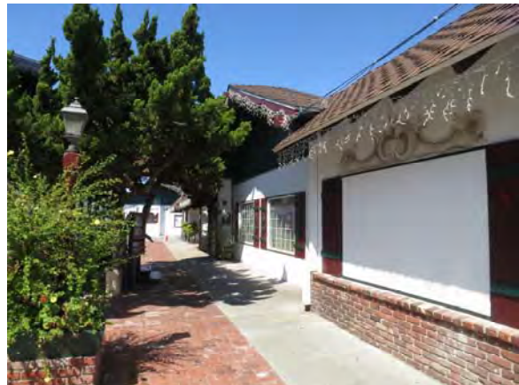
Figure 26. Infilled window at east end of south façade of Building 1.
