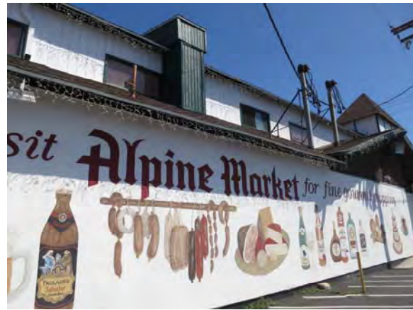
Figure 105. Mural on west façade of Alpine Market looking southeast.
