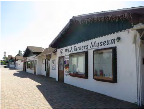
Figure 15. North façade of Building 1 looking southeast.
