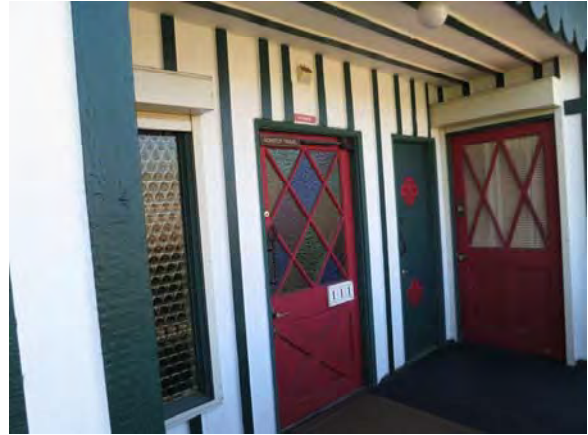
Figure 66. Door and window on second story of Building 2.
