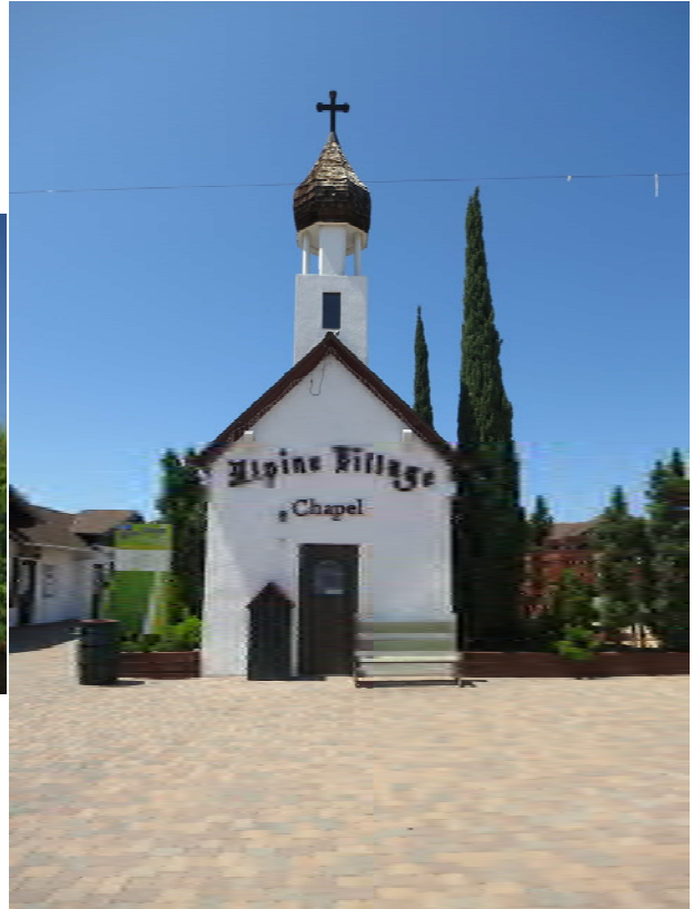
Figure 88. View of east façade of Chapel looking west.
