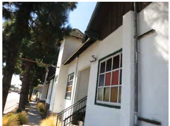
Figure 45. South façade of Building 2 looking west.
