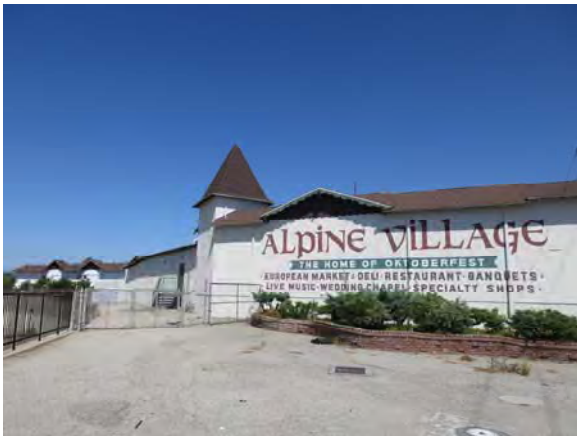
Figure 48. West façade of Building 2 looking northeast.
