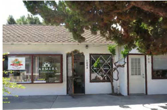
Figure 61. Insurance office on north façade of Building 2.
