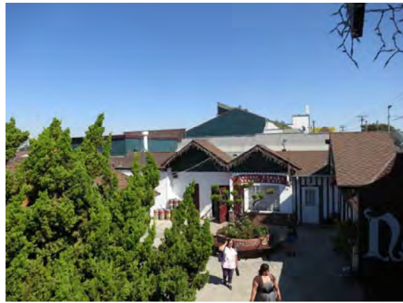
Figure 55. Same view of south end of east wing of Building 2 today.
