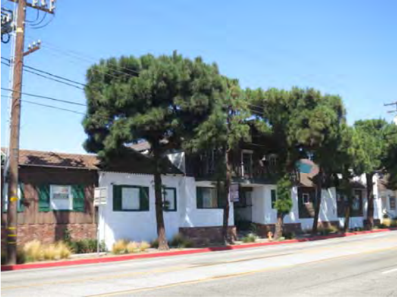
Figure 34. View of south façade of Building 2 looking northeast on Torrance Boulevard.
