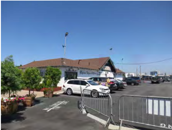
Figure 85. East façade of Building 4 looking northwest.
