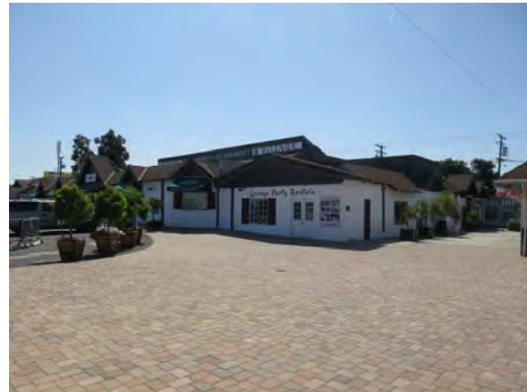
Figure 53. Oblique view showing east wing of Building 2.
