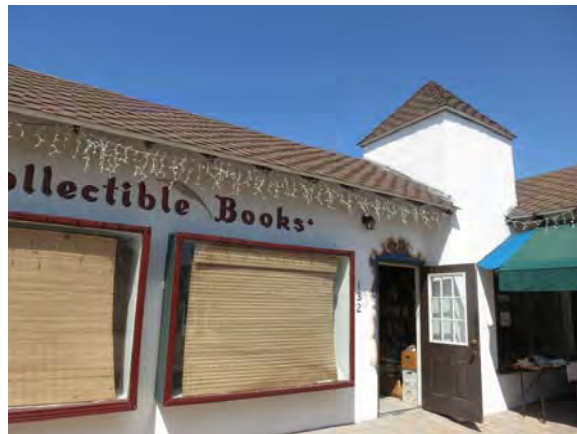
Figure 77. Detail of corner of Building 3 looking northwest.
