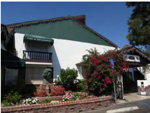
Figure 111. East façade of Alpine Inn looking northwest.
