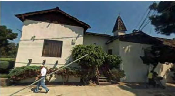
Figure 36. Google street view from 2008 showing southwest corner of Building 2.
