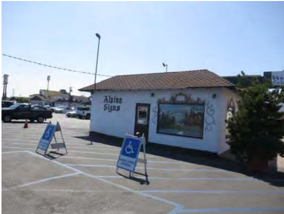
Figure 81. North façade of Building 4 looking south.
