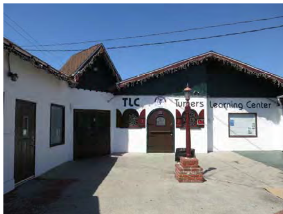
Figure 71. East façade of west wing of Building 2.
