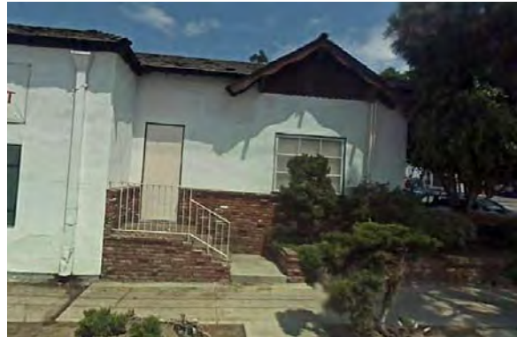
Figure 122. Google street view showing window at southeast corner, 2008.
