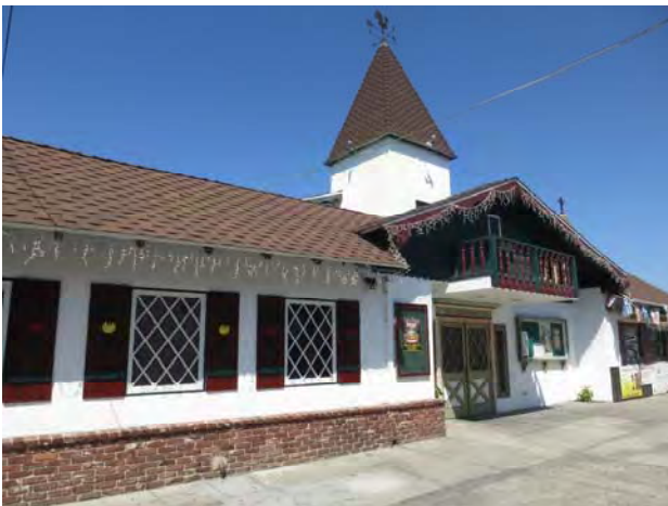
Figure 9. East façade of Building 1 looking northwest.
