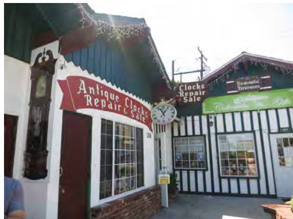
Figure 57. West façade of east wing of Building 2.
