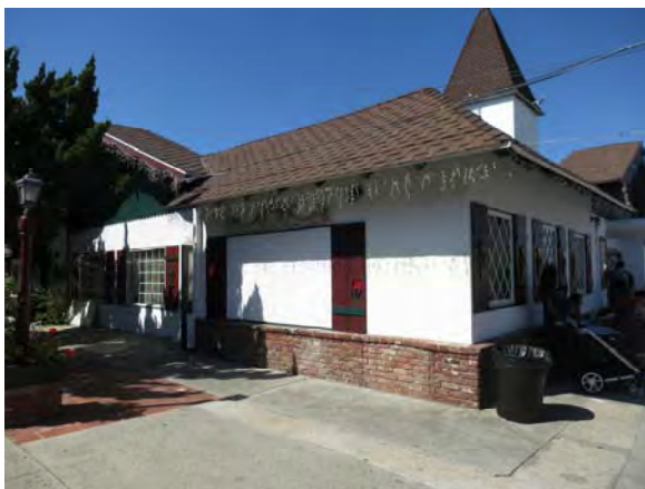
Figure 27. Wall at southeast corner of Building 1.
