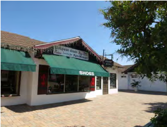
Figure 78. South façade of Building 3 looking northeast.
