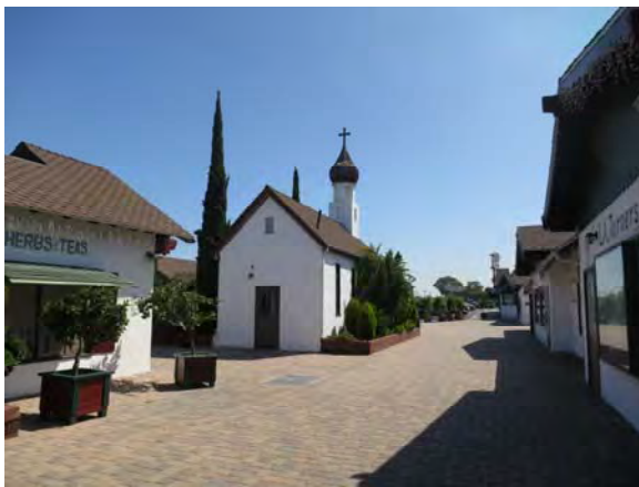
Figure 93. West façade of Chapel looking northeast.
