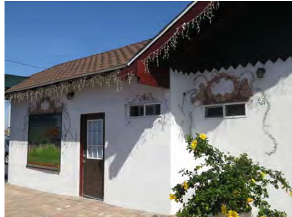
Figure 82. North end of west façade of Building 4 looking northeast.
