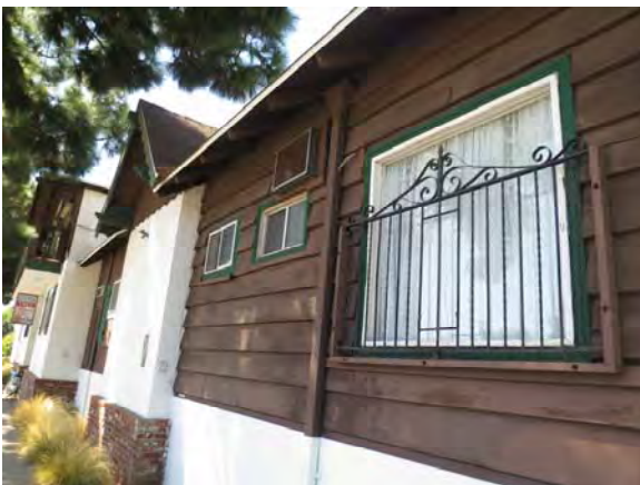
Figure 44. South façade of Building 2 showing board and batten siding.
