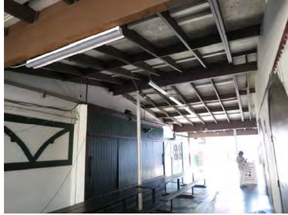
Figure 30. Covered patio looking southwest.
