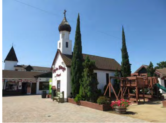
Figure 92. North façade of Chapel looking southwest.
