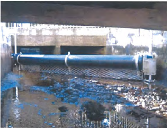
Figure 9. Bandalong Boom by Storm Water Systems. Boom comprised of an HDPE Pipe with metal mesh skirt.
