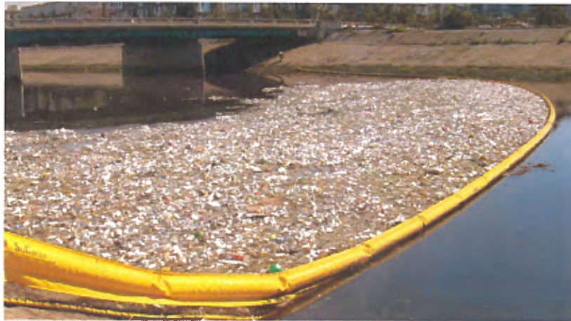
Figure 1. Ballona Creek Trash Boom (by Kepner Plastics) after a rain event.
