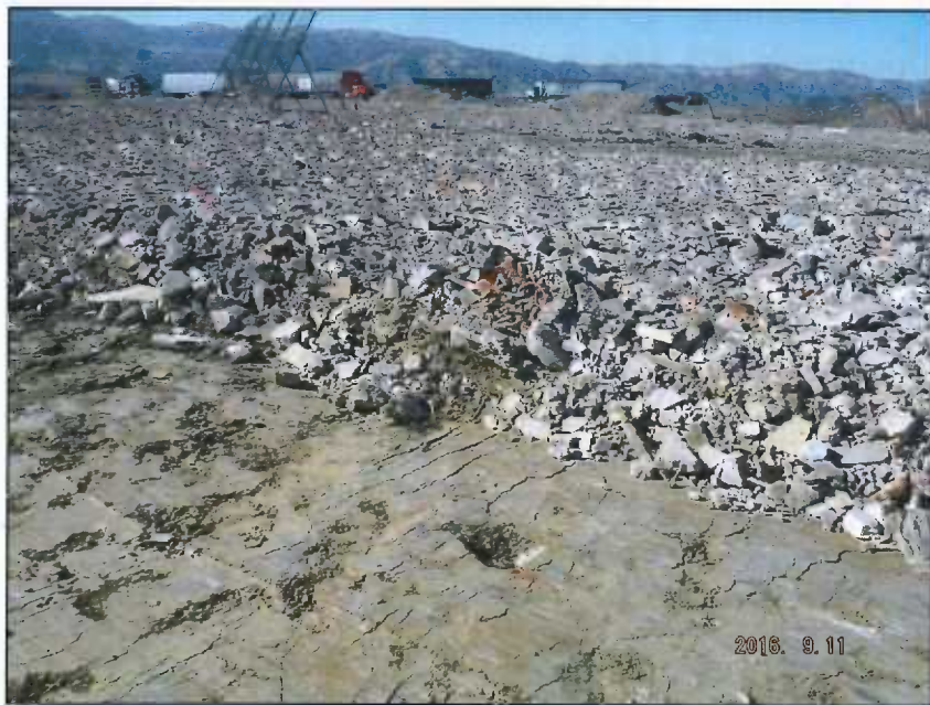
CCLF All Weather Tipping Pad – Constructed with beneficial reuse rubble
