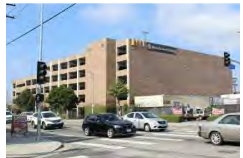
Figure 17 West Angeles Cathedral parking structure
