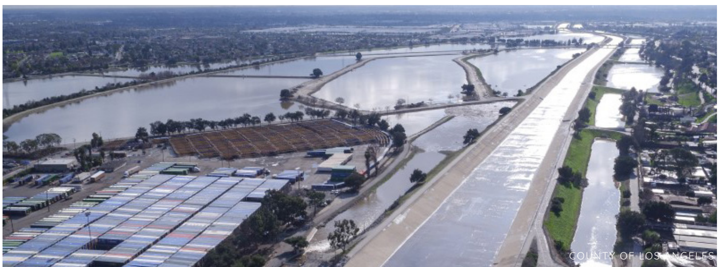
Looking downstream the Rio Hondo Channel and Spreading Grounds at the Metrolink crossing on the border of Montebello and Pico Rivera, showing high water levels after a rain and the performance of the spreading grounds in holding water and infiltrating into the ground.
