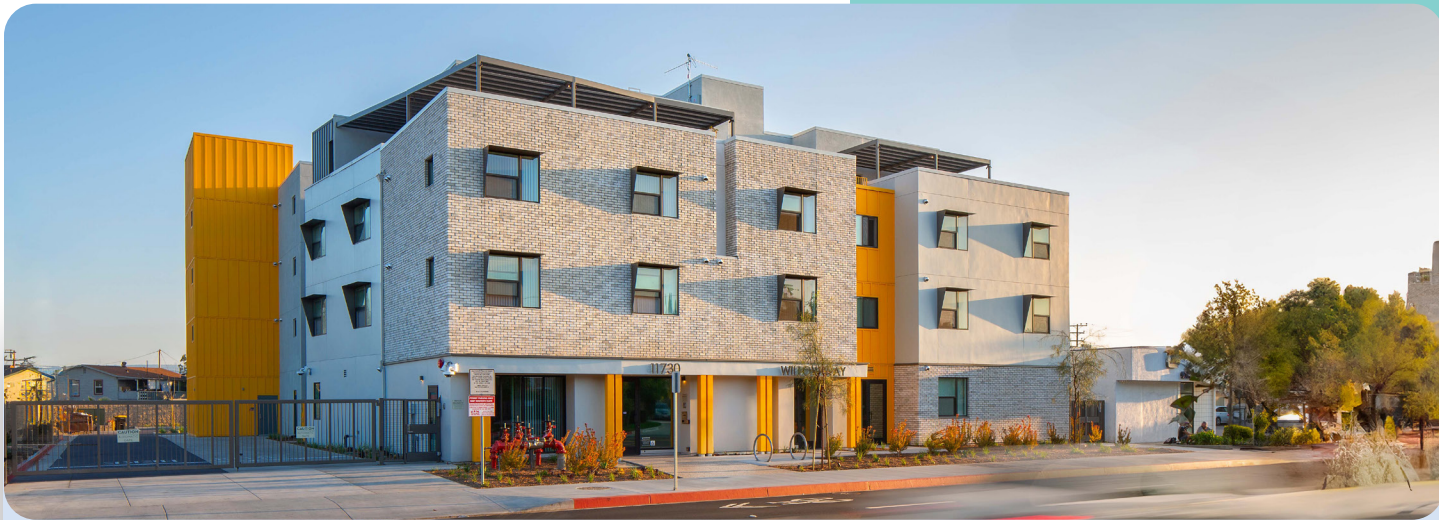
Willow Way, which includes 39 apartments, creates an opportunity for more residents to access affordable housing in the San Gabriel Valley.
