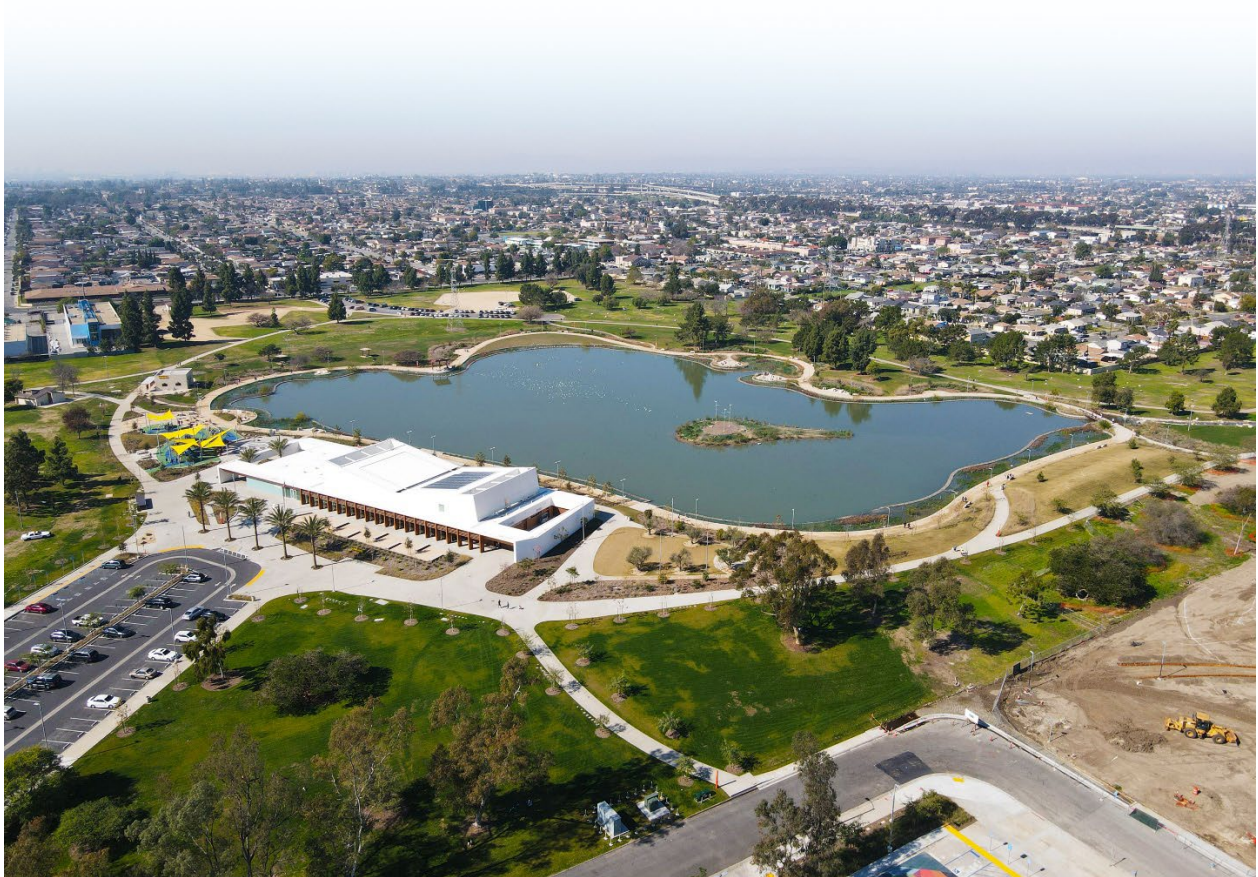
Compton Creek Stormwater and Urban Runoff Capture Project at Earvin Magic Johnson Park
