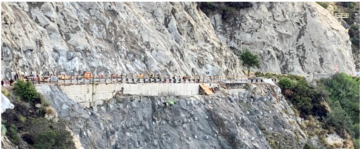
Santa Anita Dam Emergency Access Road Stabilization
