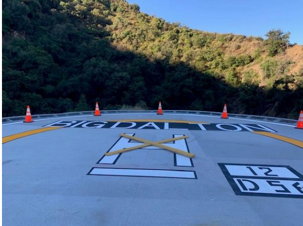
Big Dalton Dam – New Heliport
