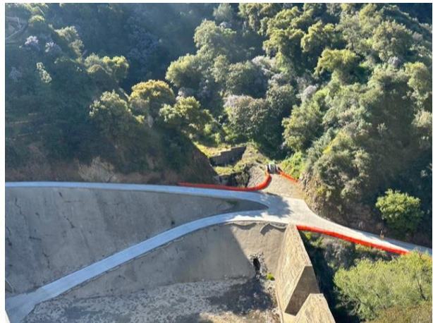
Big Dalton Dam – Access Road
