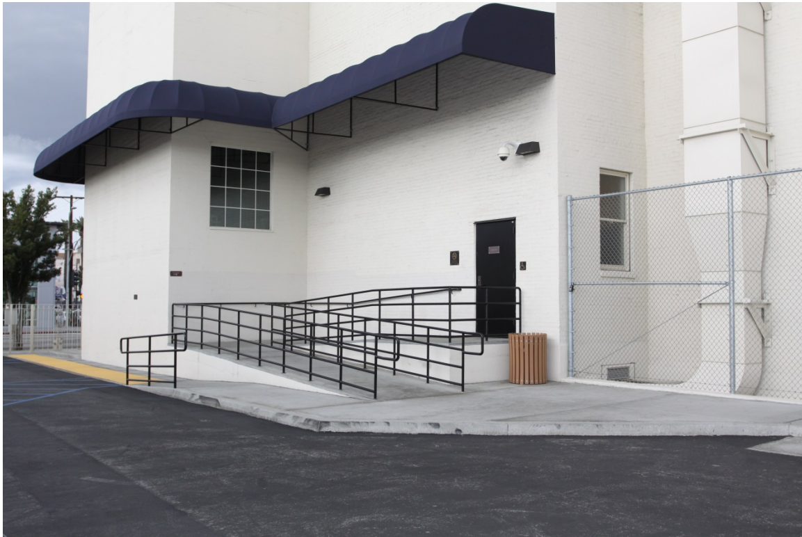
Main Entrance Wheelchair Accessible Ramp
