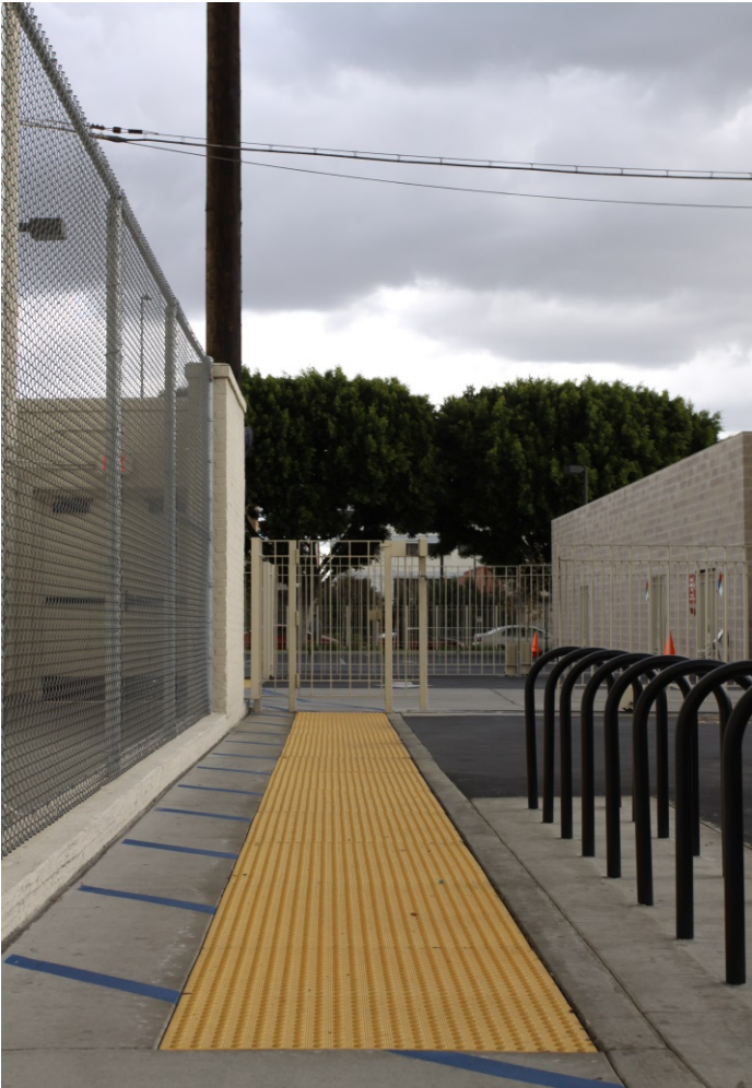
Walkway Entrance Tactical Paving Tiles
