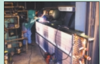
New air conditioning unit is installed at Hacienda Heights Library.
