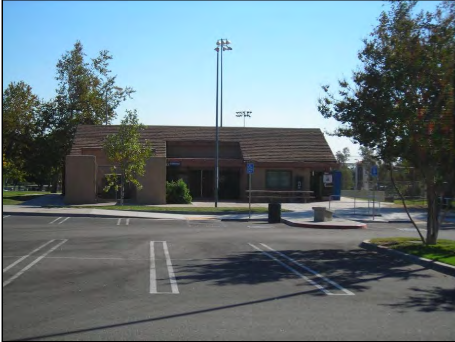
Photograph 1. Existing administration building located south of the parking lot, view to the south.
