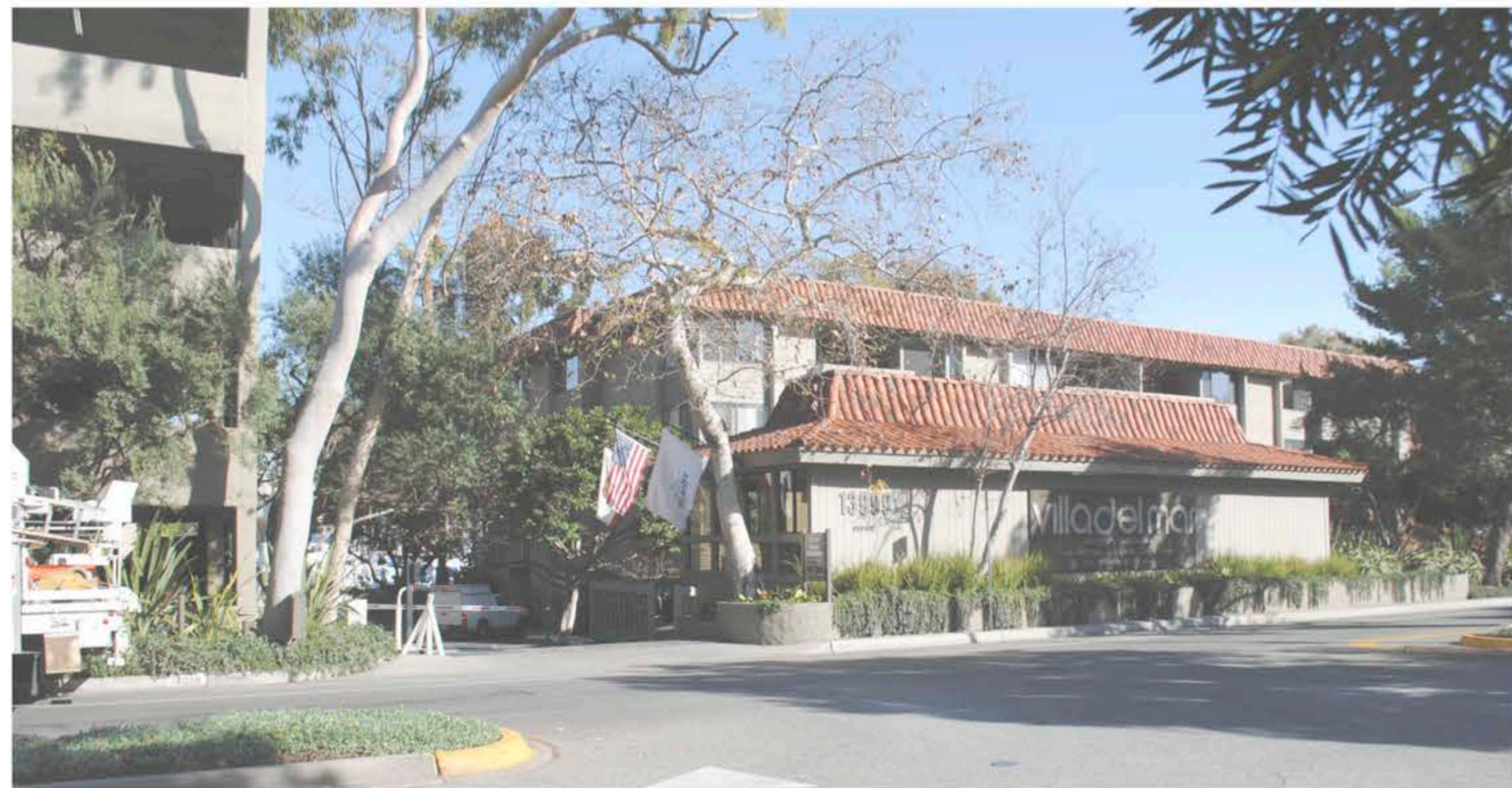
existing view of leasing office
