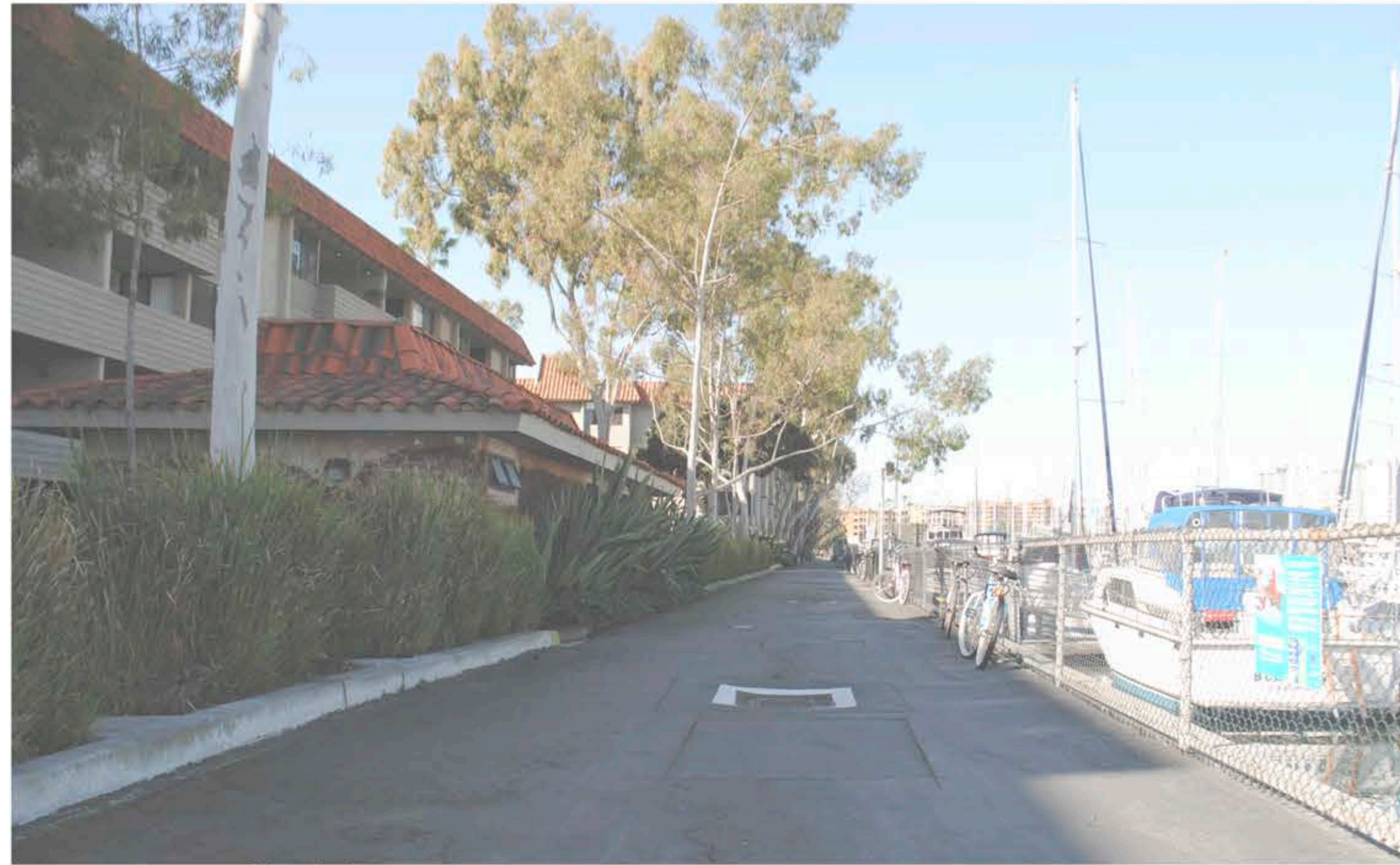
existing view of bath house
