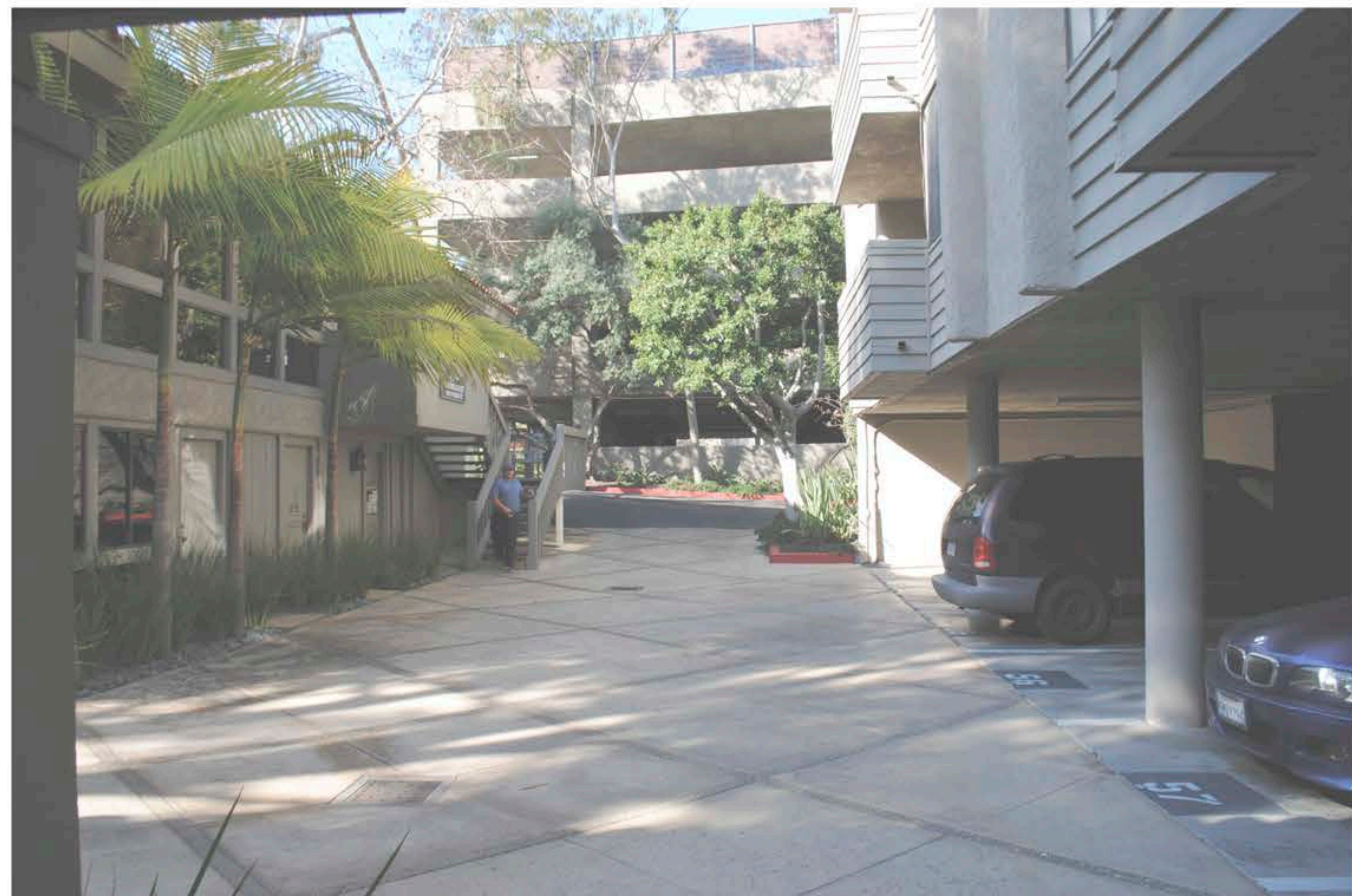
existing view of leasing court yard
