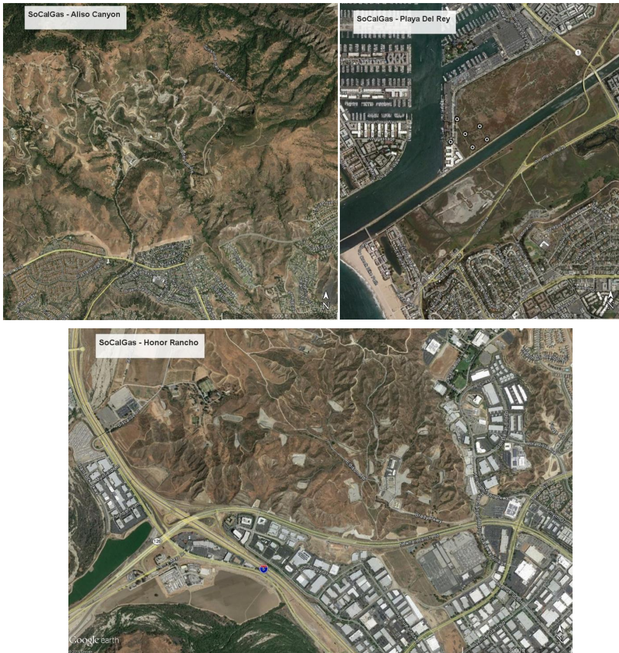
Figure 3 SoCalGas Oil Fields Aerial Overviews
