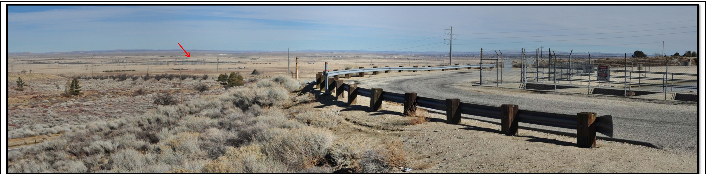
Simulation. Post-construction photographic simulation from picnic shelter along the California Aqueduct Trail in the Foothills Area.
