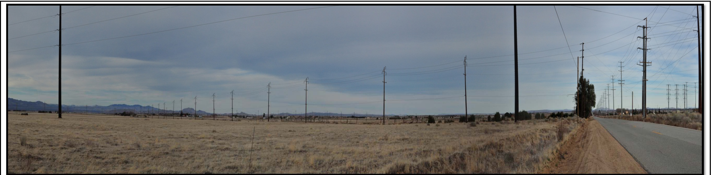
Photo 5. PP23 – Taken from eastbound West Avenue J, across the street from the Antelope Substation, approximately 0.4 miles south and 0.6 miles west of the Project Site.
