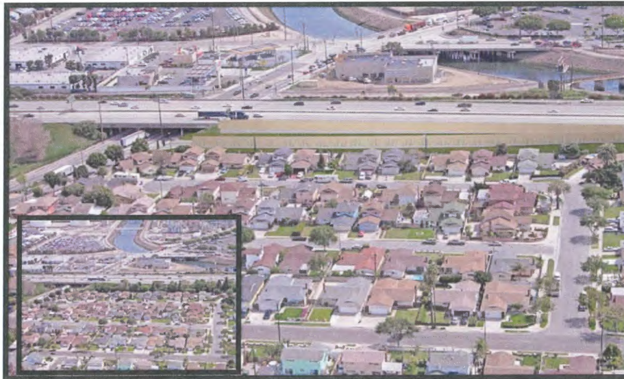
Figure 2-9 Proposed View of NB On-Ramp with Soundwalls (view looking west from the neighborhood)
