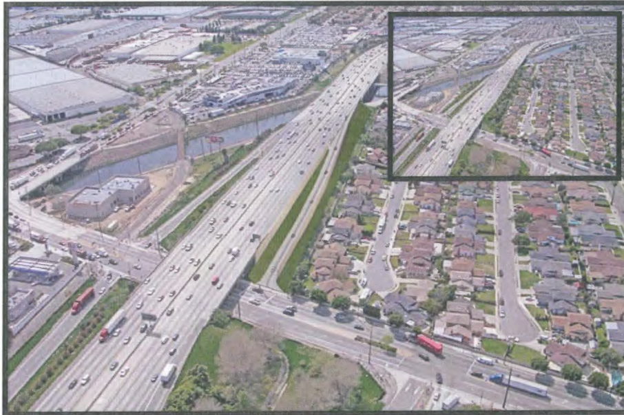
Figure 2-8 Proposed View of NB On-Ramp with Soundwalls (view looking north over the interchange)
