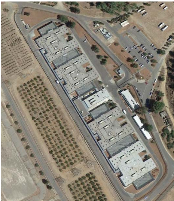
Figure 1.5: Pitchess Detention Center (North) Site
