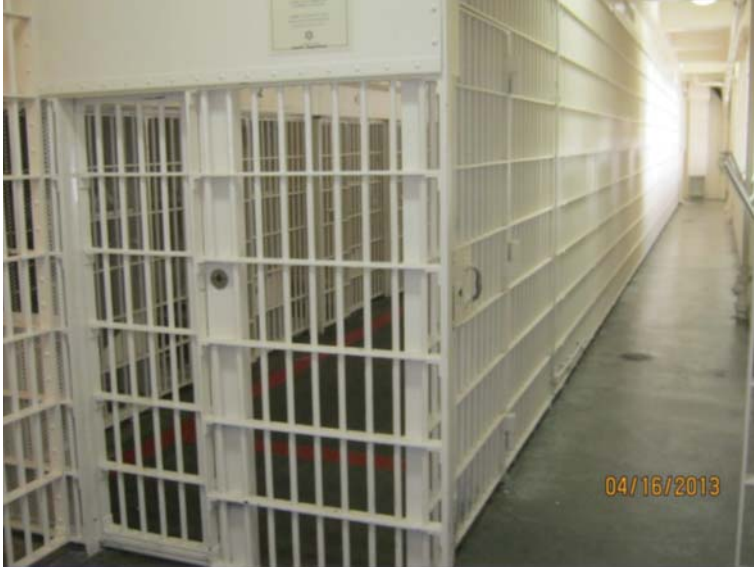
Figure 1.3: Pitchess Detention Center(East) Cell Block (Linear Design)
