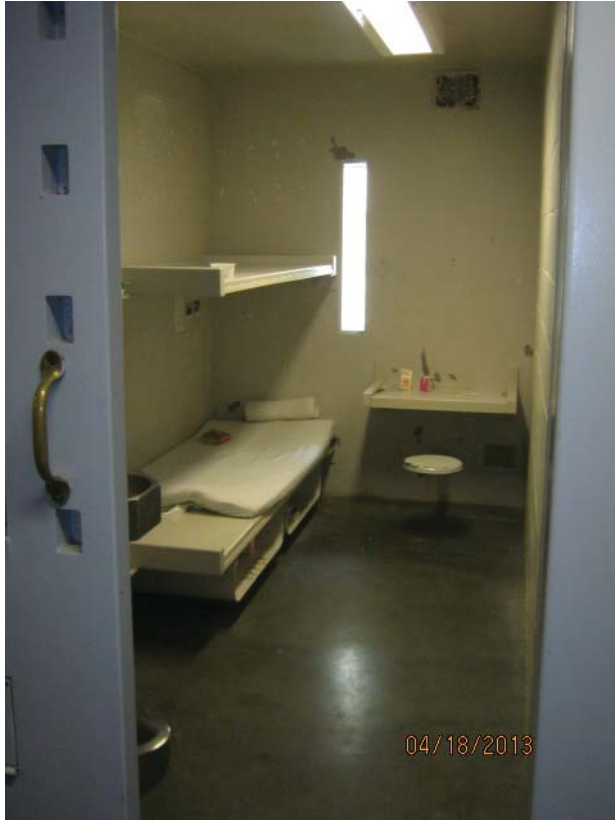
Figure 1.23: CRDF Double-Bunked Cell
