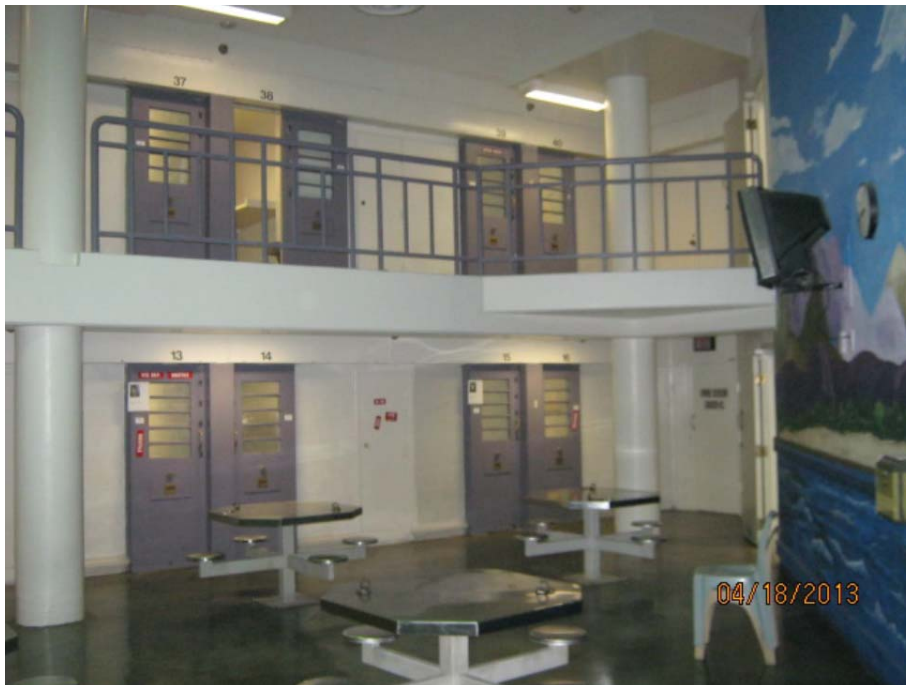
Figure 1.22: CRDF – Typical Cell Block Dayroom
