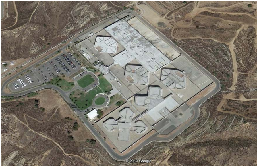
Figure 1.10: North County Correctional Facility Site
