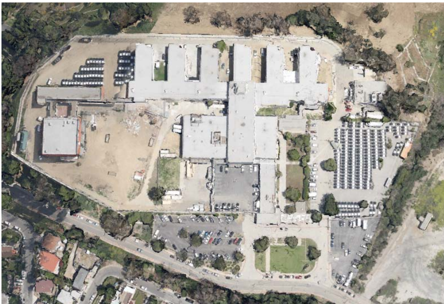
Figure 1.29: Sybil Brand Institute Site
