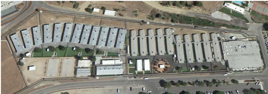
Figure 1.8: Pitchess Detention Center (South) Site
