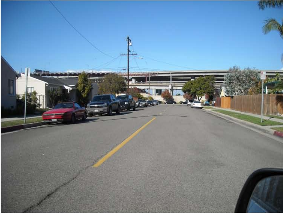
Judah Avenue viewing north - Project site is on the left and single-family residences are on the right. Metro rail line and I-105 are in the background.
