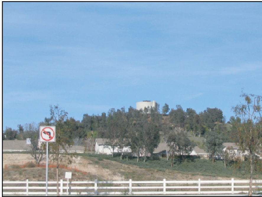
Water Tank from Newhall Ranch Road and Bridgeview Lane
