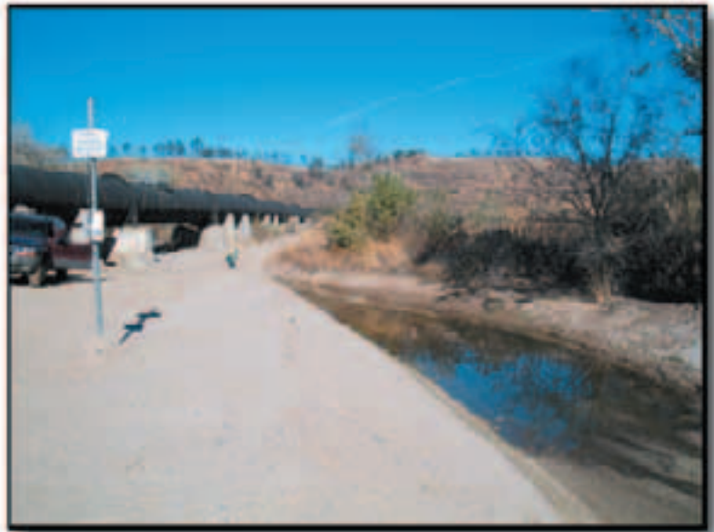
Site 2 – Sampling of DWP Aqueduct Pipeline Crossing on South Bank
