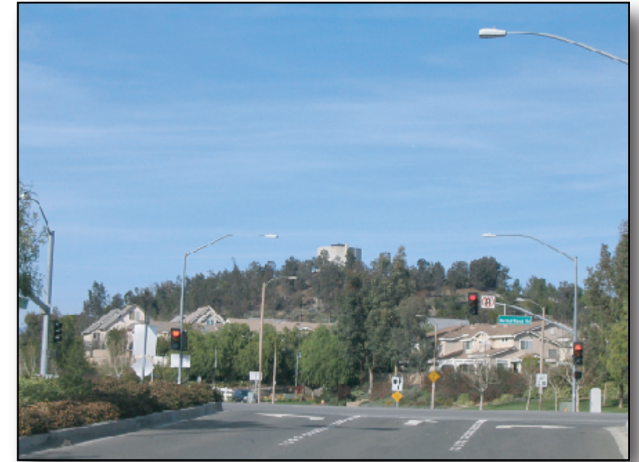
Water Tank from Newhall Ranch Road and Grandview Drive
