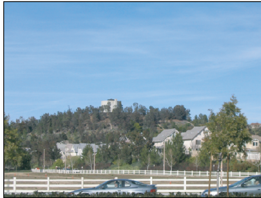
Water Tank from Newhall Ranch Road West of Grandview Drive
