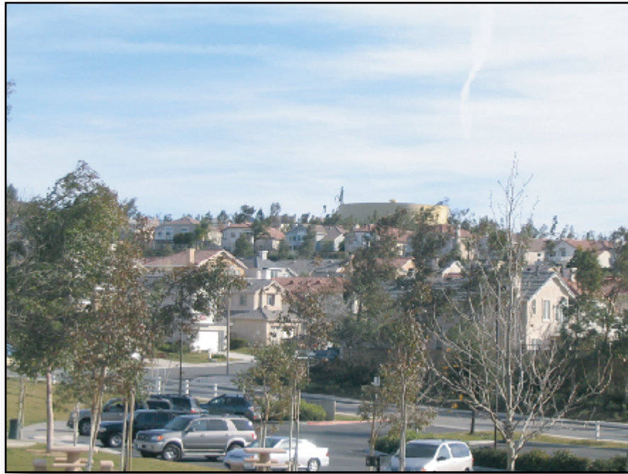
North Park Water Tank from McBean Parkway Pedestrian Bridge
