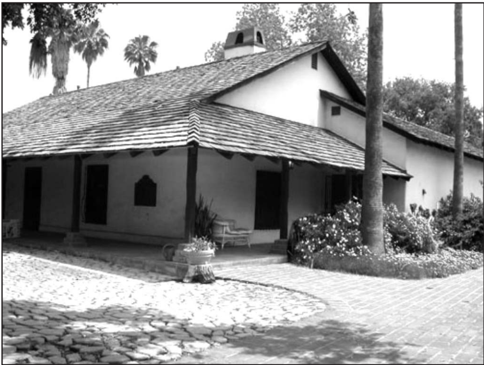
View of the Ortega-Vigare Adobe from Ramona Street.
