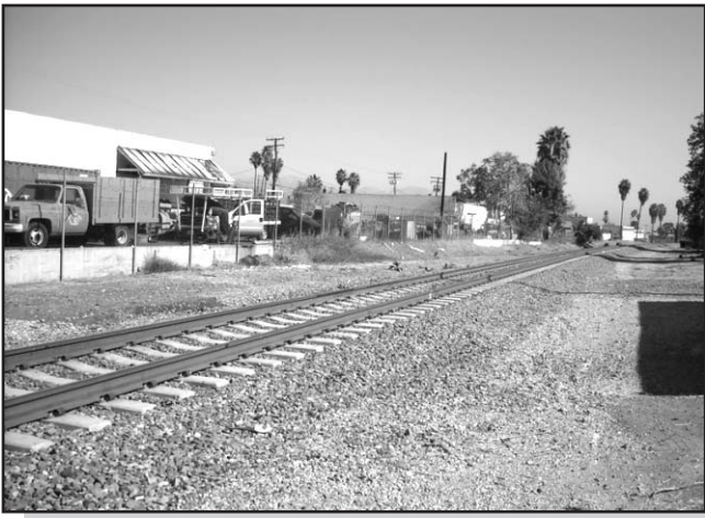
Project site looking east from Del Mar Avenue.
