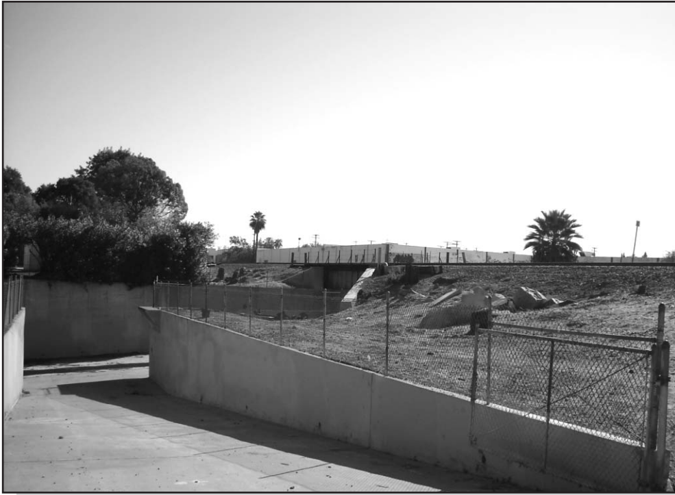
Looking southeast, from a stormwater ramp at the end of Commercial Avenue, towards the existing Union Pacific Railroad bridge over the Rubio Wash.
