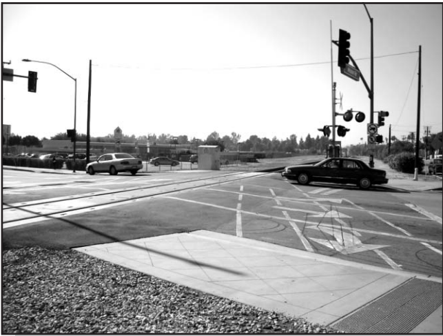
Looking west at the existing Ramona Street crossing.
