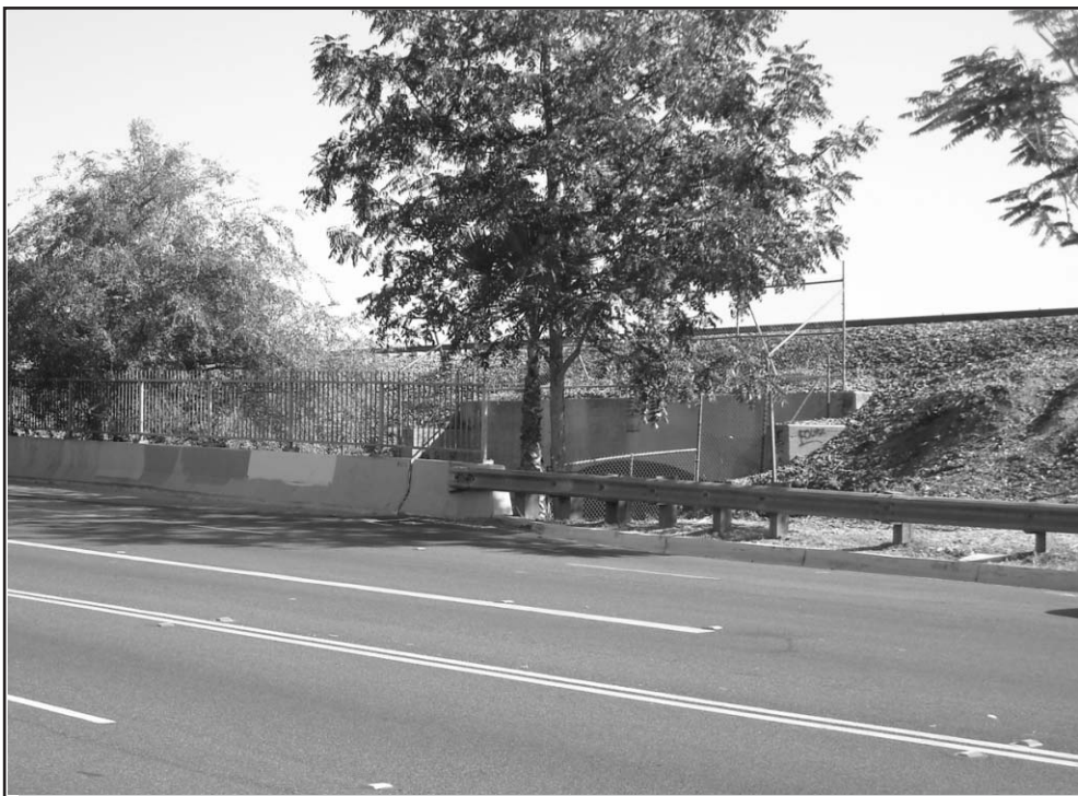
Looking southeast towards the existing Union Pacific Railroad bridge over the Alhambra Wash, adjacent to Mission Road.
