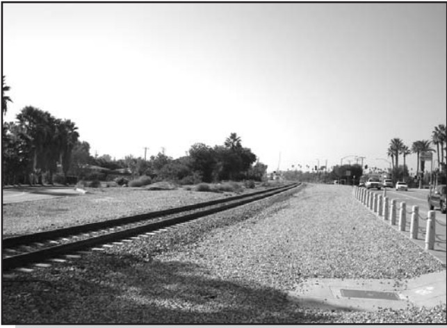
Project site looking west from Mission Road.
