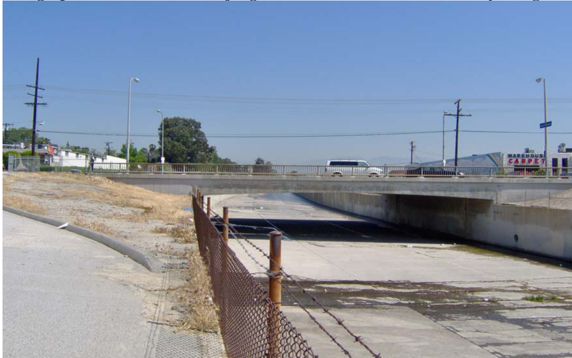
Photograph 8: View north on Tujunga Wash centered on Sherman Way Bridge
