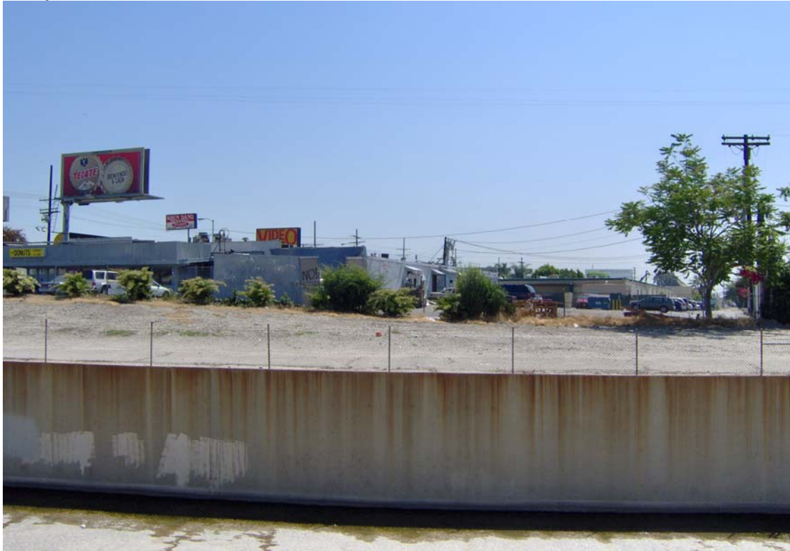
Photograph 7: Tujunga Wash channel with view of east side 70' ROW backed by strip commercial development along Sherman Way, NHO in the San Fernando Valley
