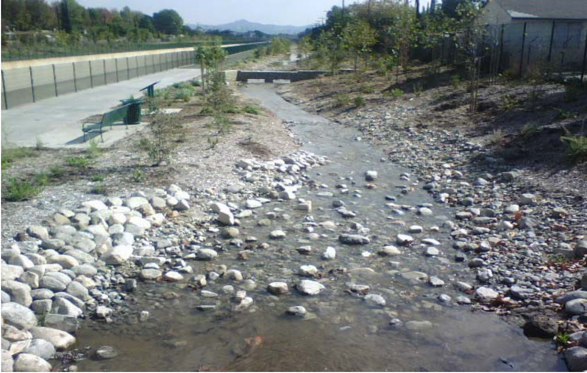
Photograph 5: L.A. County Department of Public Works Downstream Project
