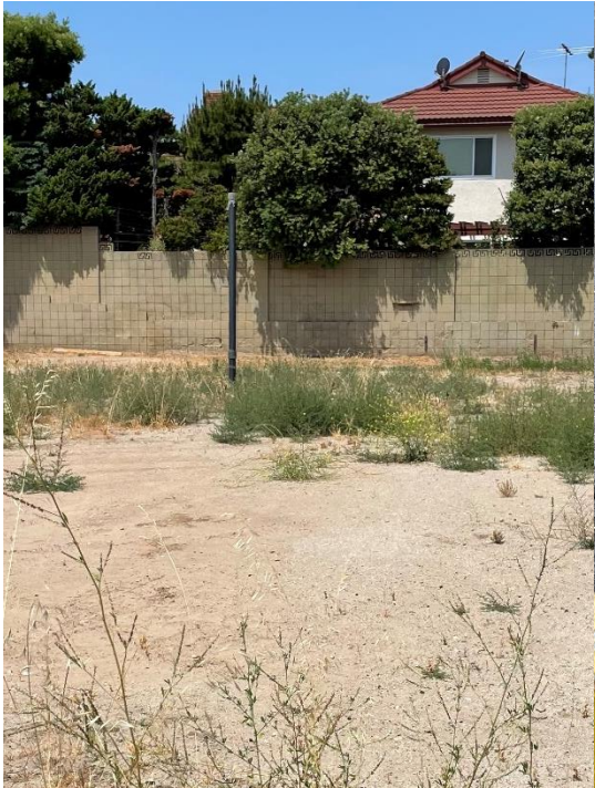
Abandoned well vent cone
