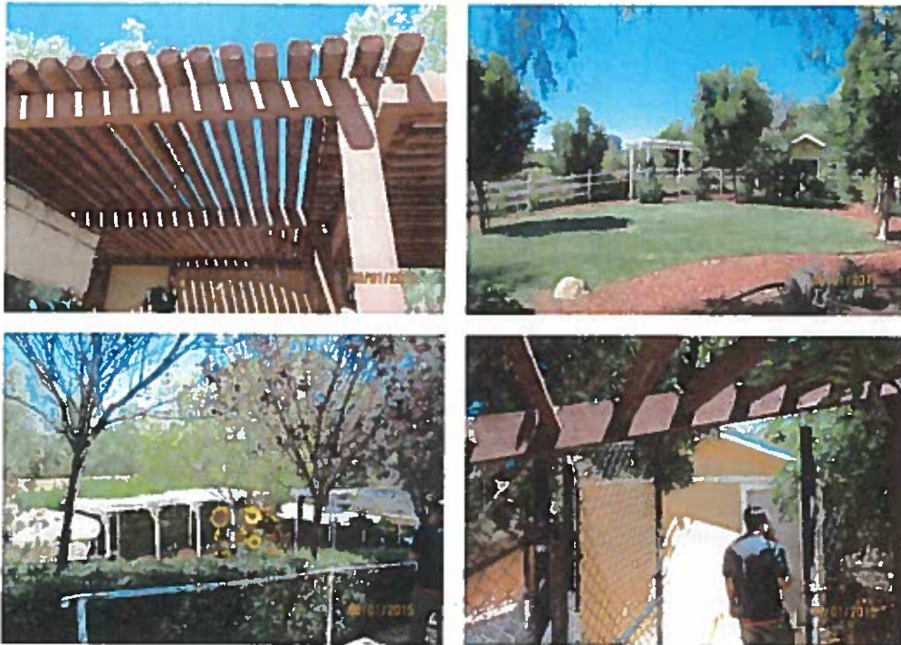
Figure 2: Structures not depicted in the approved Exhibit "A" site plan of CUP 00-082
