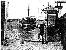
A portable boom system is used to divert runoff to the vacuum suction device so as to prevent wastewater from entering storm drains.
