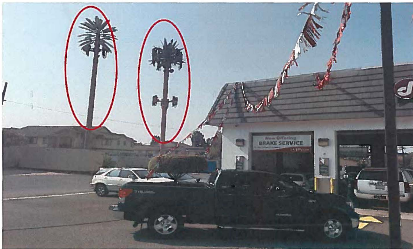
2 WTF Palm Monopine Located at Jiffy Lube
