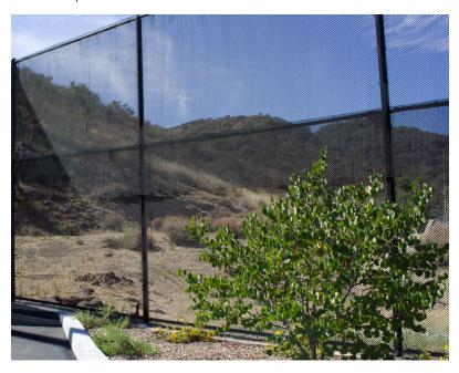
The fence fabric used is a ¾" woven wire fabric with a black coating. This fabric was not available in full height mesh so there is an approximate lap of 24" horizontally around the entire perimeter. Existing galvanized posts and rails were field painted black to match the fabric color. In corners
