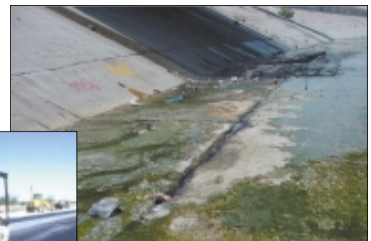
Flood Control Channel cleaning.
