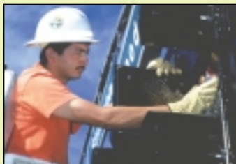
Traffic Signal relamping.
