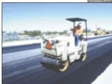
Road Maintenance working on a road improvement project
