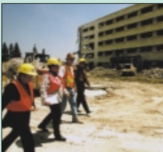
An AA team conducts an on-site inspection.
