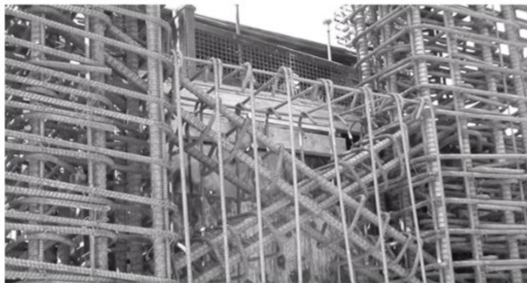
Figure 2. Typical diagonally-reinforced concrete coupling beam with full confinement.
