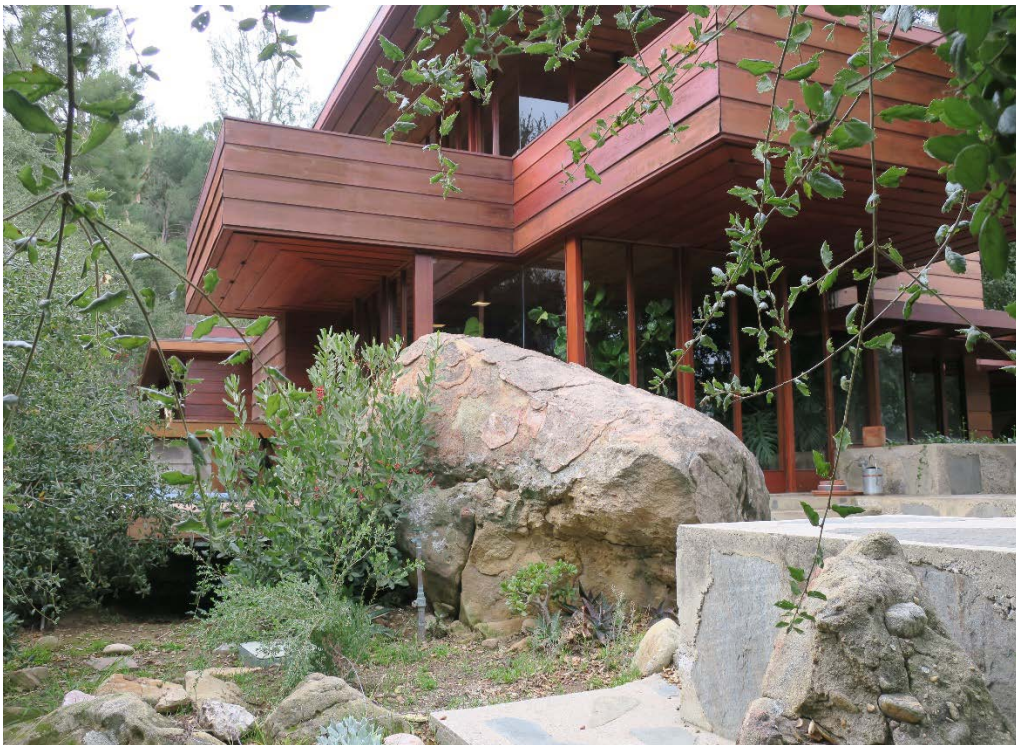
View west of the east façade and second story balconies. Note the original concrete/stone paving in the foreground (ARG, 2019).
