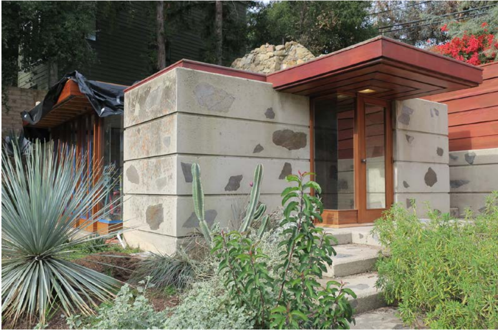
View north of the utility shop's east and south façades (ARG, 2019).
