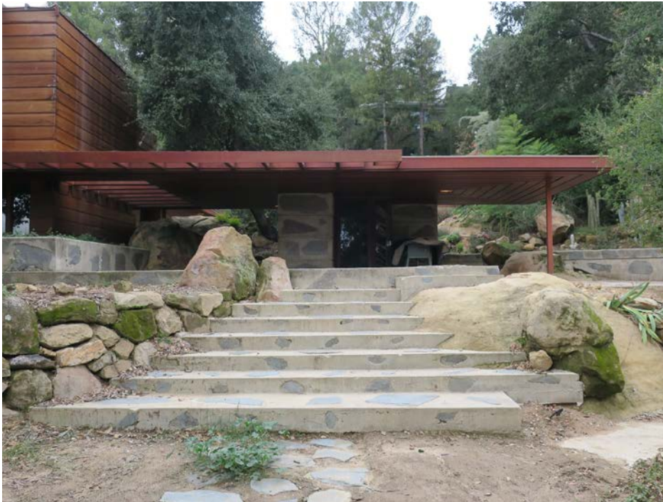
View west of the carport/entrance canopy and concrete steps with embedded stone (ARG, 2019).
