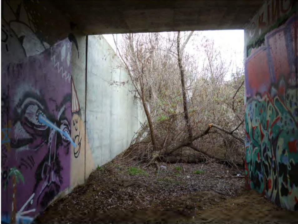
Figure 3-4 Invert in West Barrel of Triple Box Culvert Under 101 Freeway
