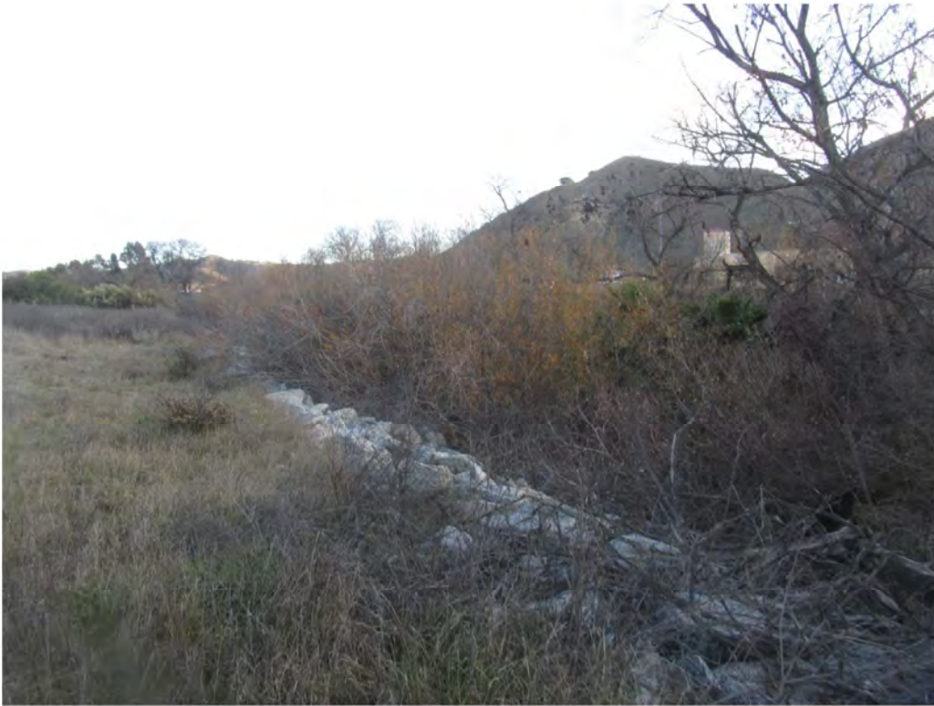
Photograph 7- Las Virgenes Creek north (upstream) of the open culvert with rip rap stabilized banks.
