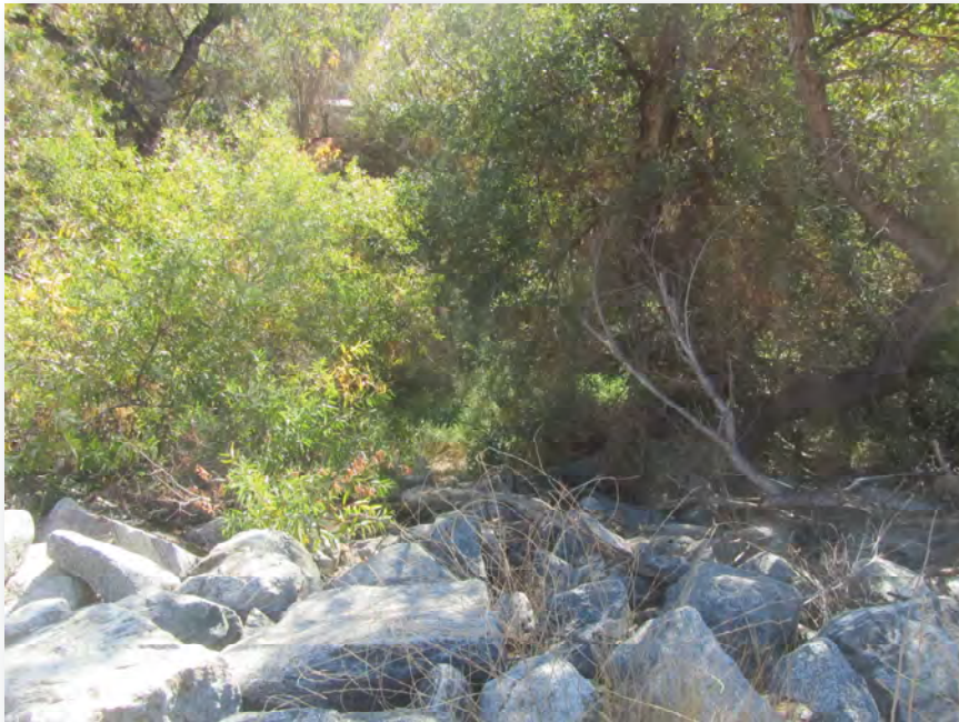
14. View of riprap looking north from concrete channel.
