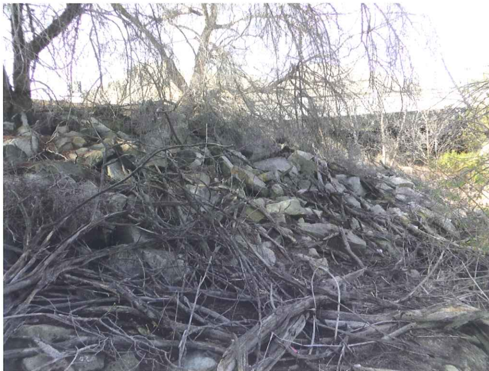
Photograph 7- Western bank of Las Virgenes Creek stabilized by riprap.
