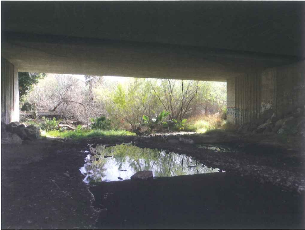
Photograph 1- Heavily disturbed area under the Agoura Road Bridge.
