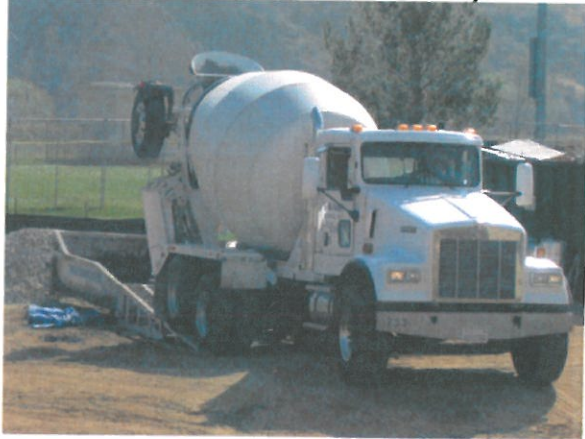
Collect Concrete Washout & Recycle
