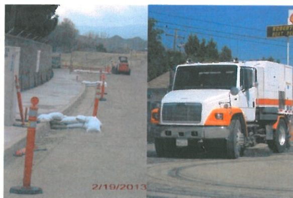
Gravel Bag Berm & Sweeping for Sediment Control on Street
