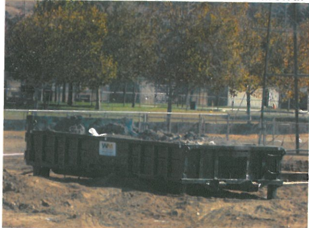
Recycle Concrete Debris to Base Material
