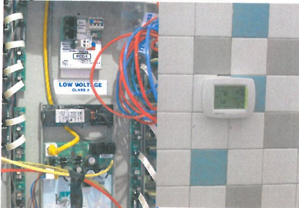
Lighting Central Control Panel & Programed HVAC Thermostat
