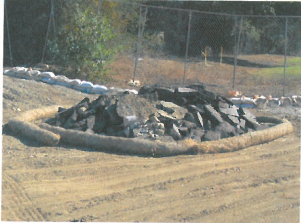
Recycle Asphalt Debris to Base Material
