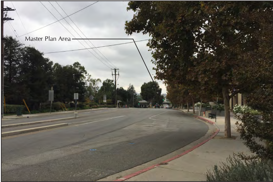
PHOTO 7 Horse Lane Trail - October 27, 2019 Facing West-Northwest
