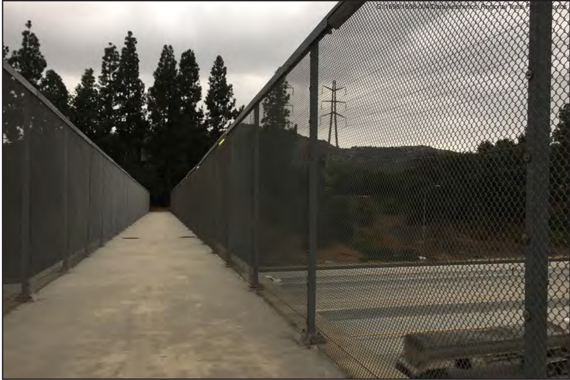
PHOTO 1 Horse Lane Trail - October 27, 2019 Facing West-Northwest
