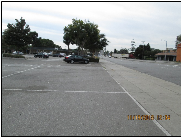
(Photo 8) Western boundary – View south along Pioneer Boulevard
