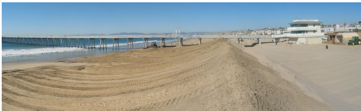
Figure 14. Construction of temporary winter sand berm at Hermosa Beach. The berm protects the lifeguard headquarters building public beach asset. The County's winter berm program is effective as a relatively low cost measure to protect landward facilities from high tides and moderate storm wave runup. The berms are maintained as needed throughout the winter season by the Department of Beaches and Harbors.
