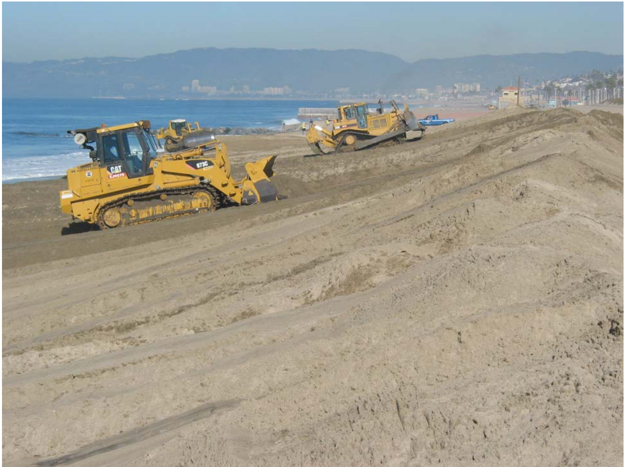
Figure 5 Typical Winter Sand Berm Construction
