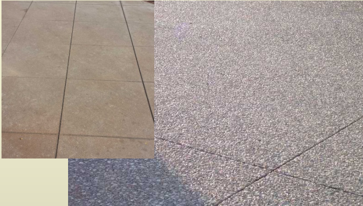
Exposed Aggregate Concrete Paving
