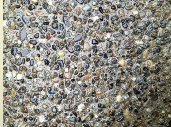
Seeded Concrete Band w/ Crushed Aggregate
