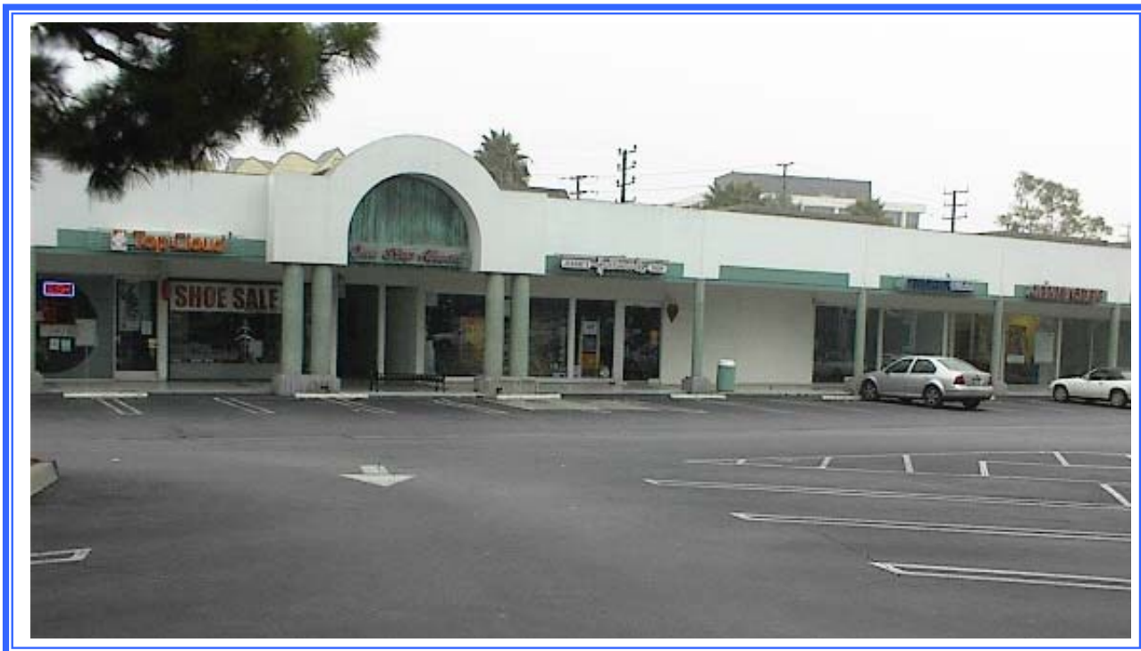
Waterside Shopping Center - Parcel 50 Before
