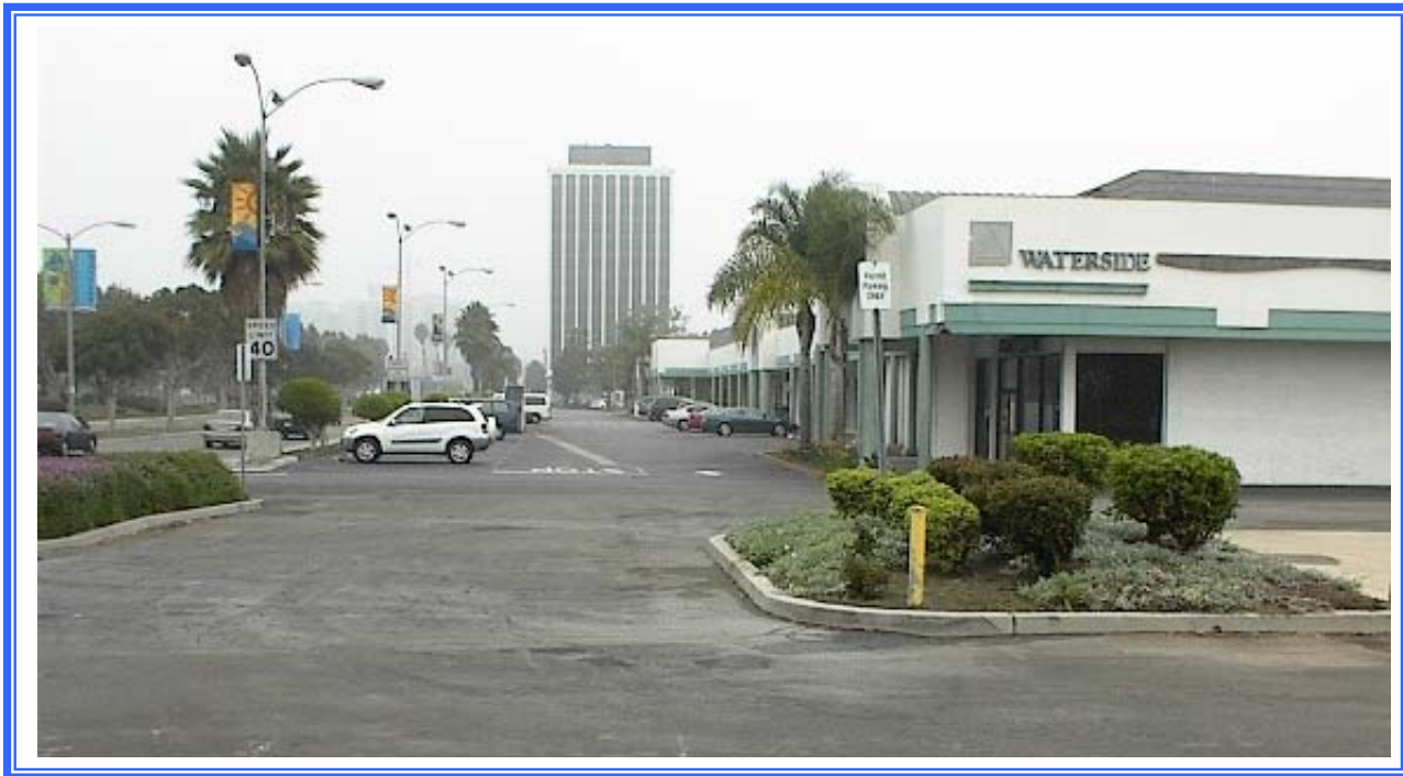
Waterside Shopping Center - Parcel 50 Before
