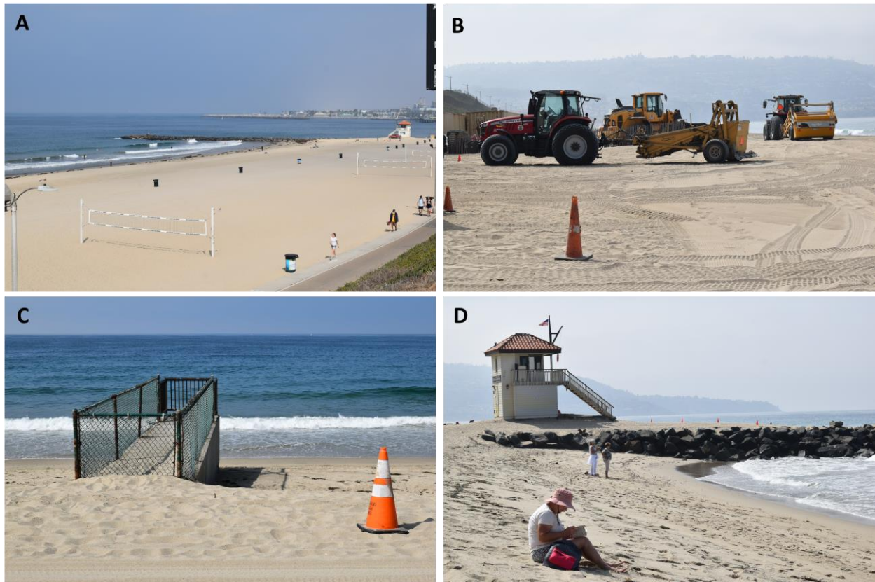
Figure 23. South Redondo Beach Existing Condition Photos (Taken Oct 5th, 2022): A. Overview With Volleyball Courts, Lifeguard Tower, And Groin, B. Sand Moving Equipment, C. Cross-Shore Structure, D. Groin With Typical Downdrift Accretion/Updrift Erosion Response
