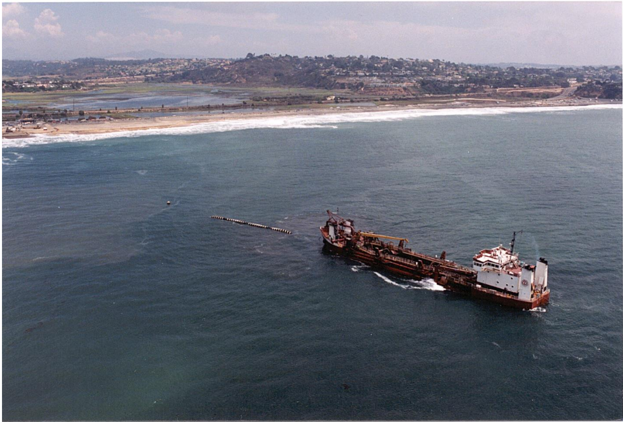
Figure 13. Hopper Dredge Pumping Sand Onto Cardiff Beach As Part Of San Diego Regional Nourishment
