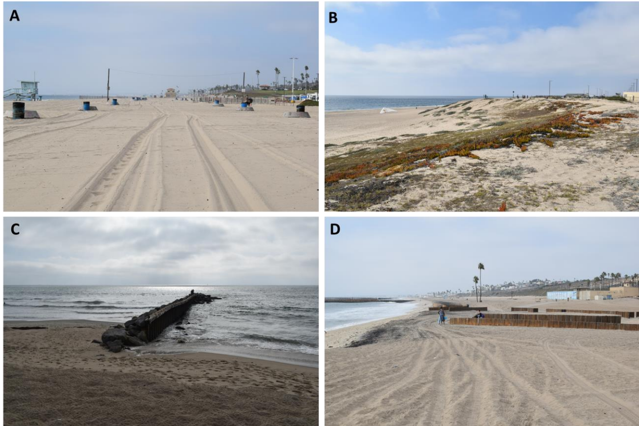
Figure 16. Dockweiler Beach Existing Condition Photos (Taken Oct 5th, 2022): A Wide Beach Berm With Fire Pits, B Vegetated Dunes Used For Paragliding, C Sheet Pile Groin With Typical Downdrift Accretion/Updrift Erosion Response, D ADA Access
