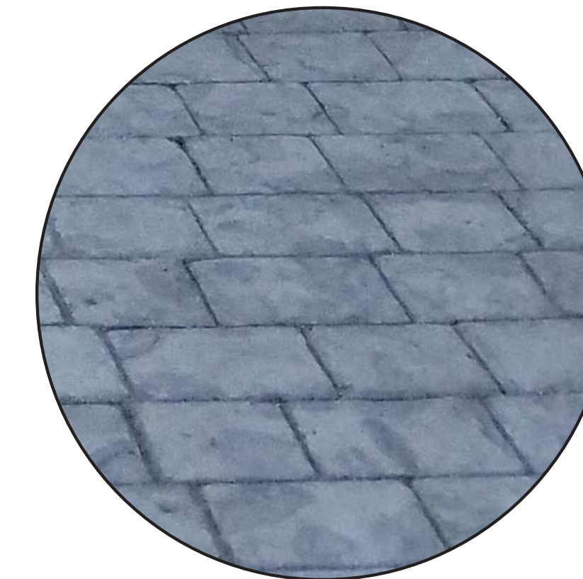
12 ACCENT PAVING - EXISTING CONCRETE PAVERS TO BE SANDED
