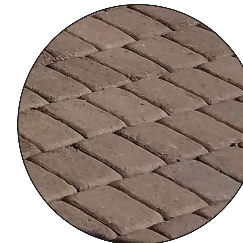
13 ACCENT PAVING - EXISTING CONCRETE PAVERS TO BE SANDED
