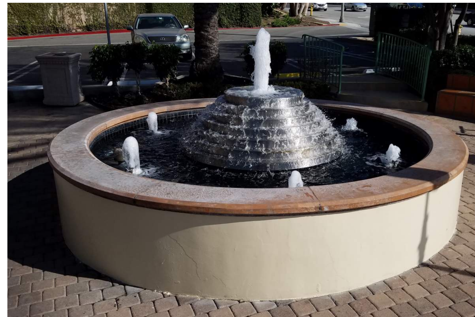
2 FOUNTAIN 'SHROUD' ENCLOSURE - ALUMINUM WITH FAUX HOT ROLLED STEEL FINISH
