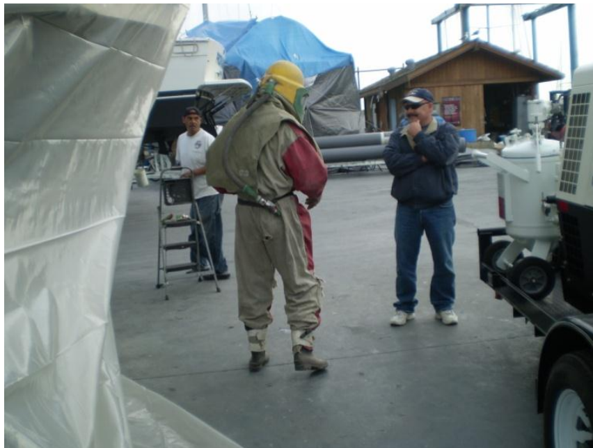
Figure 4-7. Sodium Bicarbonate Stripping Vendor Preparing to Strip Boat
