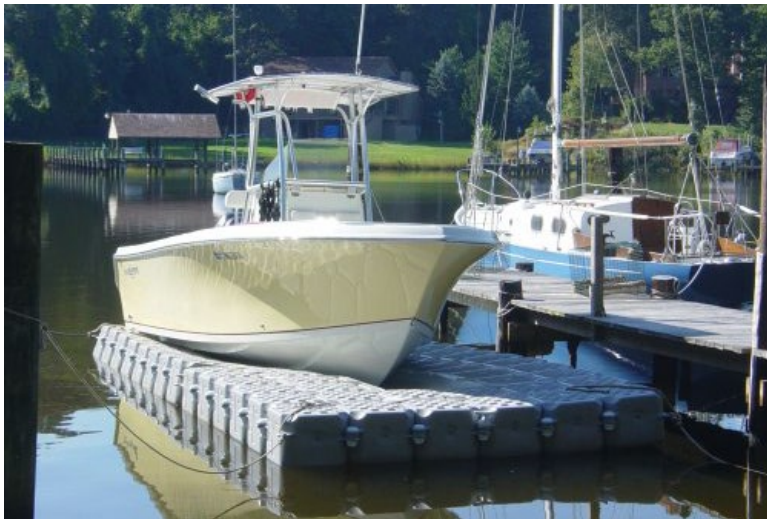
Figure 7 Picture of floating cube system R
