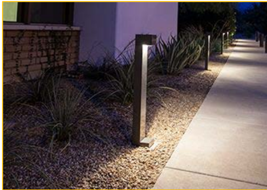
Pedestrian-oriented bollard lights
