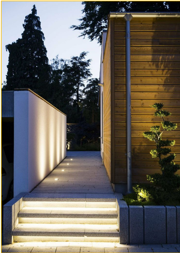
Integrated lighting in building exterior
