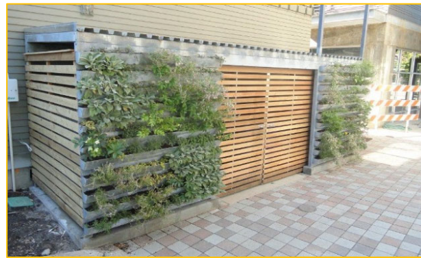
Screened trash enclosure
