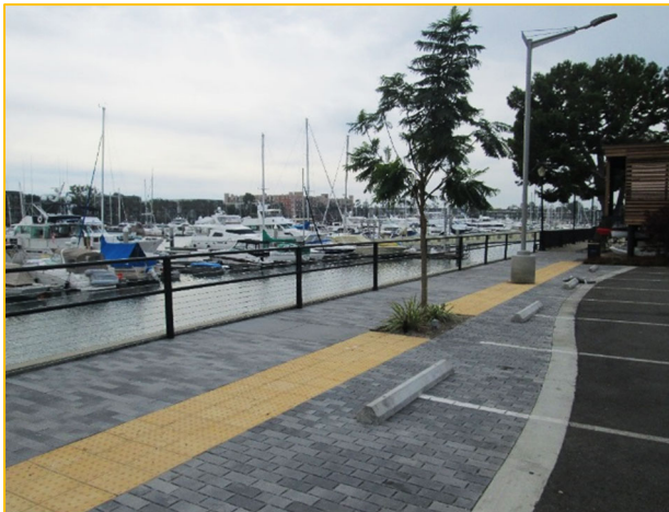
Parking lot permeable pavers, Marina del Rey
