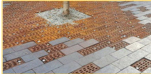
Permeable Paving
