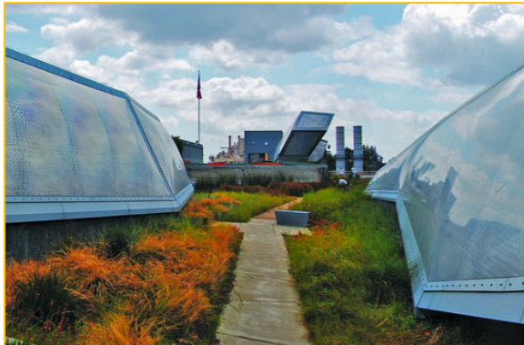
Green roof - Art Center College of Design, Pasadena
