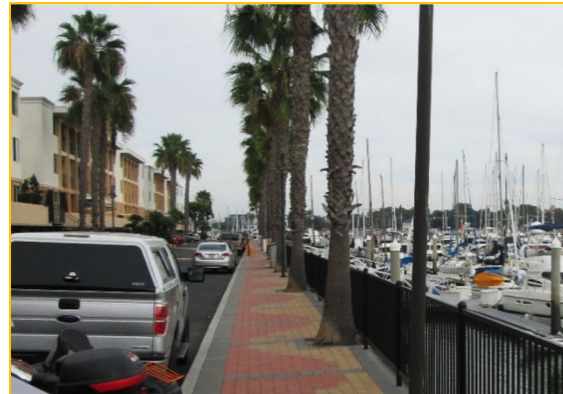
Palm trees planted too close to the seawall
