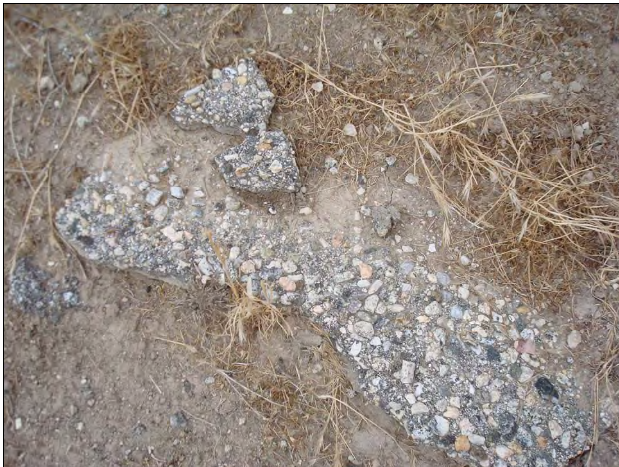
Photo 5. Typical Broken Asphaltic Concrete Surface Material on Subject Property
