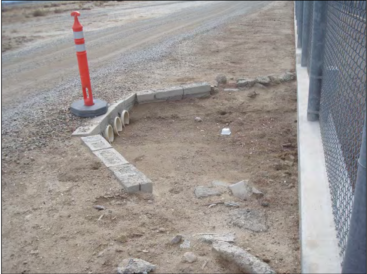
Photo 8. Drainage Swale on Northwest Portion of Subject Property
