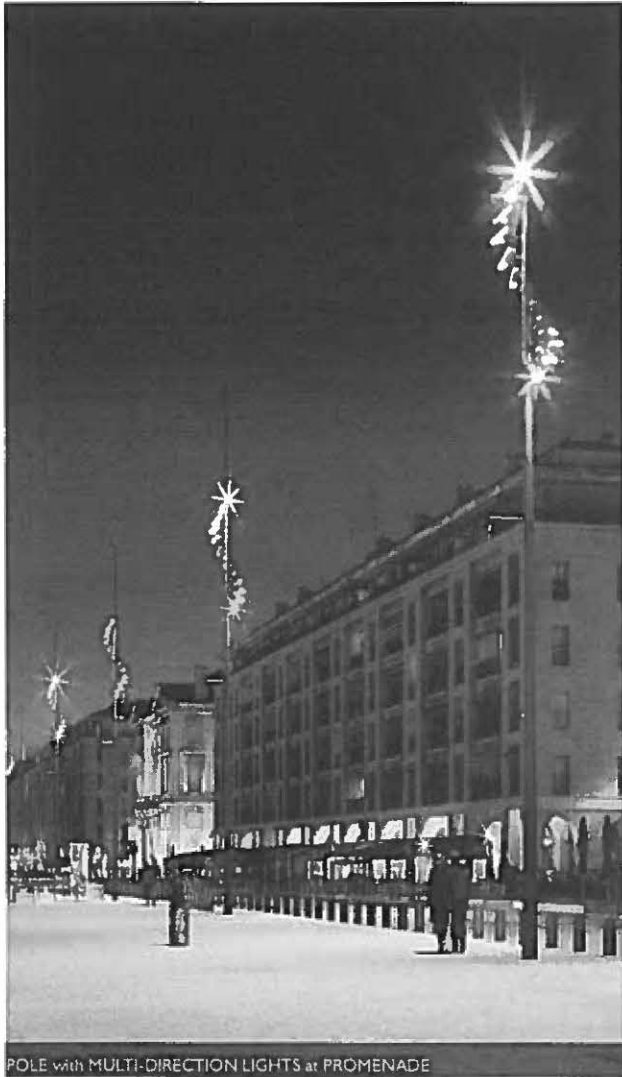
POLE with MULTI-DIRECTION LIGHTS at PROMENADE
